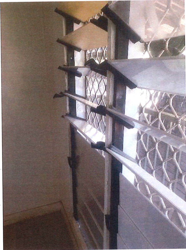
New Louvres and Galleries throughout
