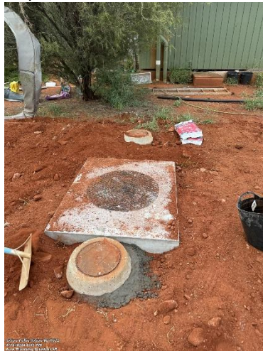
Septic Remediation Works:
