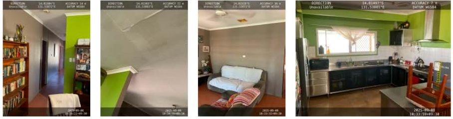
Interior existing conditions
