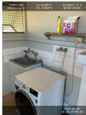
Replacement of the sink tap with a new tap.
