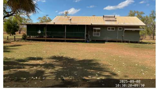
Exterior existing conditions
