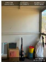
Laundry area Supply and install new enclosed shelves for the storage of all laundry materials and cleaing equipments
