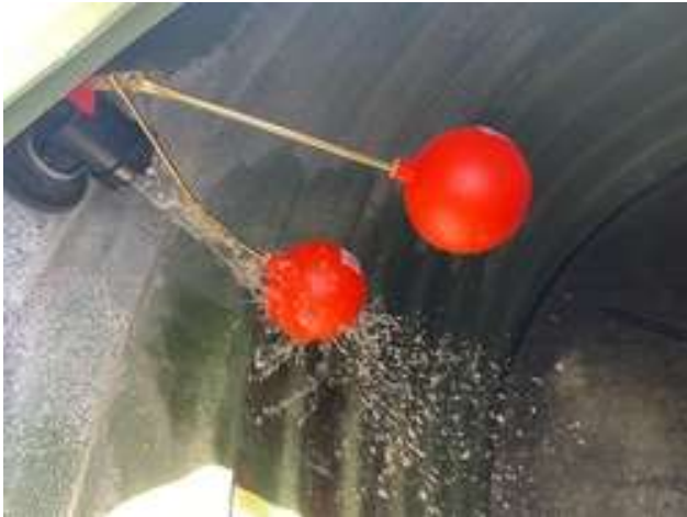
Water reinstated to over tank and house
