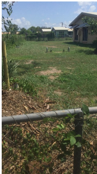
Figure 7 Water meter (lot), condition: good
