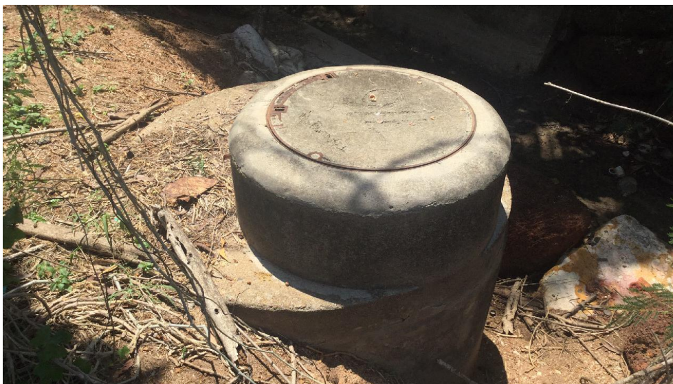
Figure 1 Sewer manhole, condition: very good
