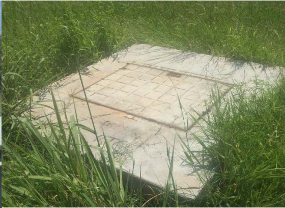
Figure 2 Sewer manhole, condition: very good
