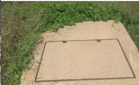
Figure 3 Sewer manhole, condition: very good
