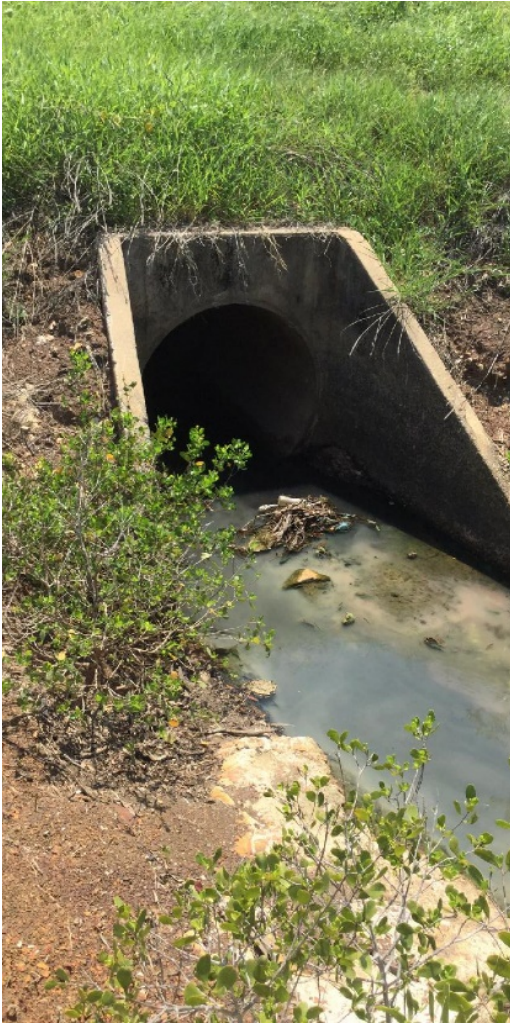
Figure 12 Headwall
