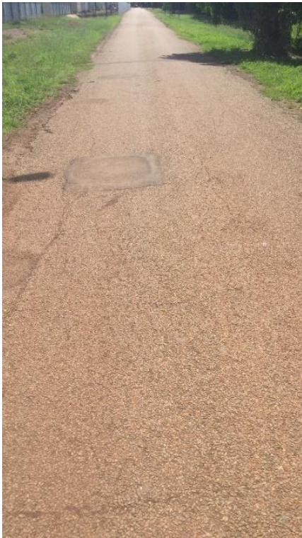
Figure 6 Pavement, condition: good
