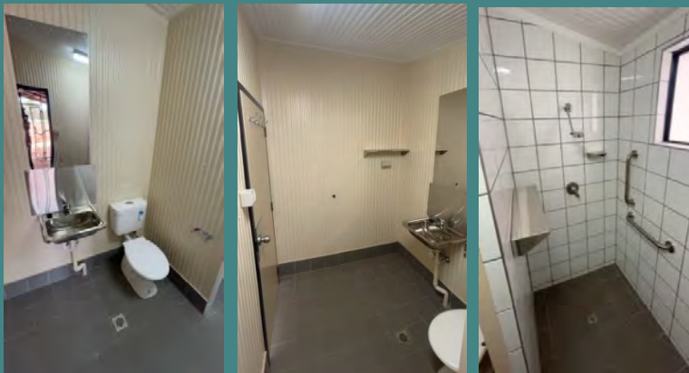
After Bathroom & Toilet works commenced:
