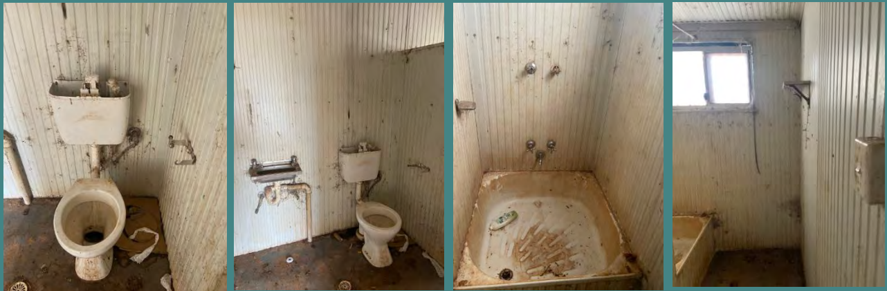
Before Bathroom & Toilet works commenced:
