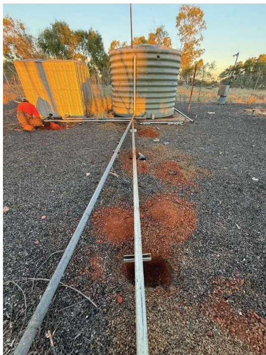
Installation of above ground pipe work
