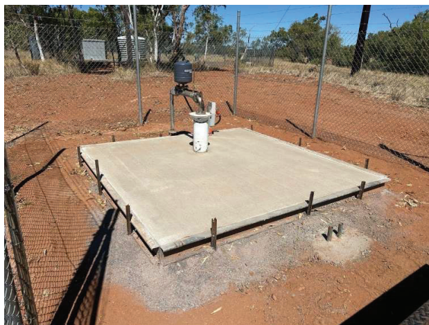
Formwork to be removed
