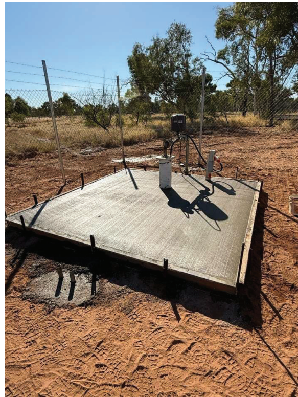
Formwork removed and stone spread
