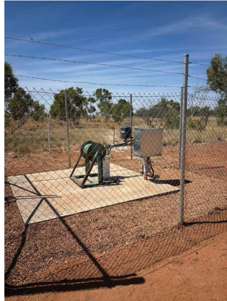
Control panel install project complete
