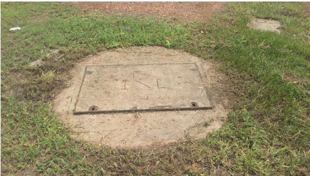
Figure 2 Sewer manhole (good condition)
