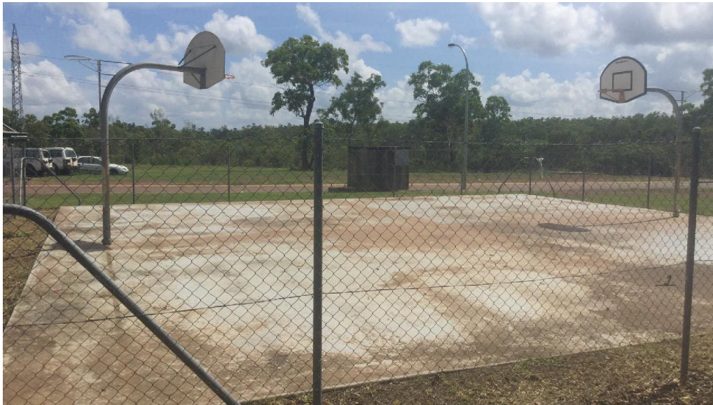
Figure 15 Basketball court, condition: good
