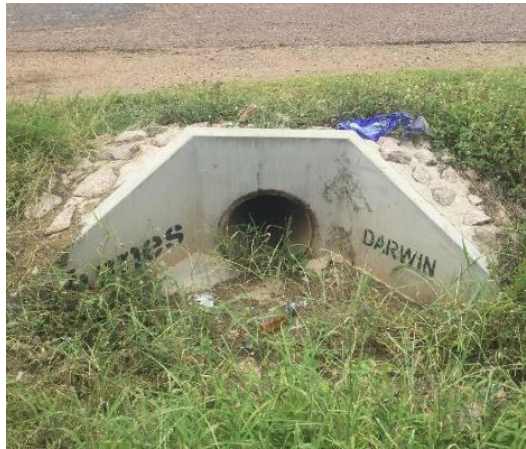
Figure 14 Headwall DN375, condition: very good
