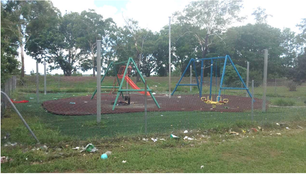
Figure 16 Playground, condition: poor
