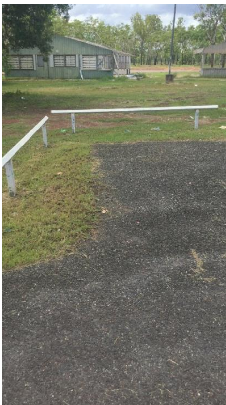
Figure 7 Carpark, condition: good
