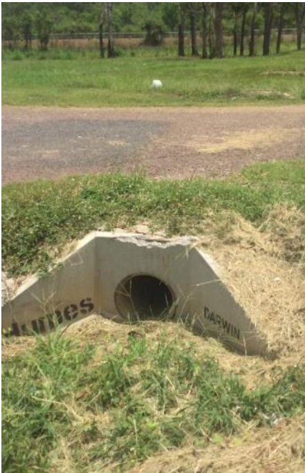
Figure 13 Headwall DN375, condition: good
