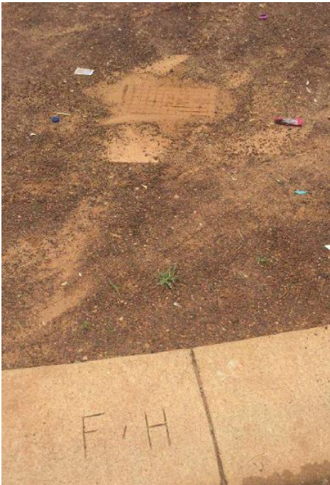
Figure 4 Fire hydrant, condition: good
