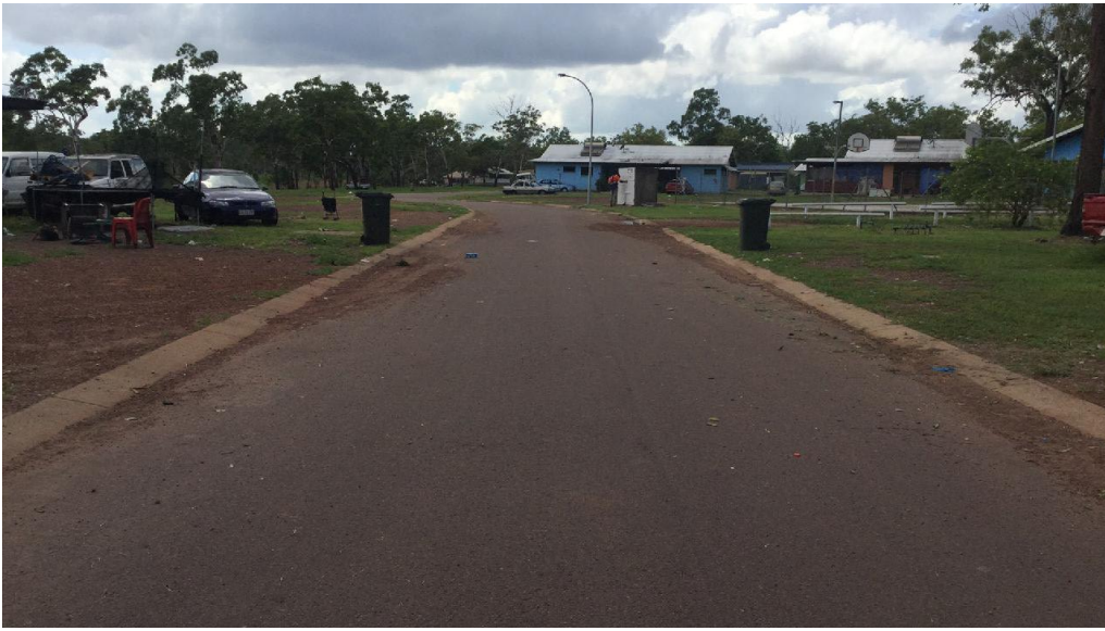
Figure 9 Pavement, condition: good
