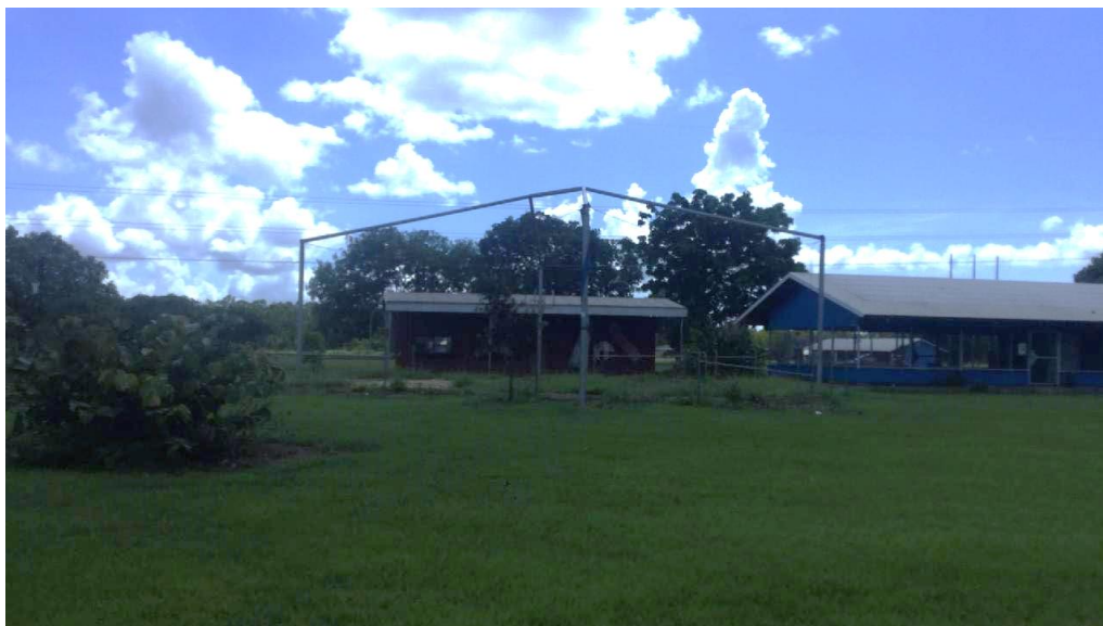
Figure 10 Playground, condition: very poor
