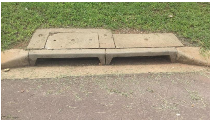
Figure 12 Side entry pit, condition: good
