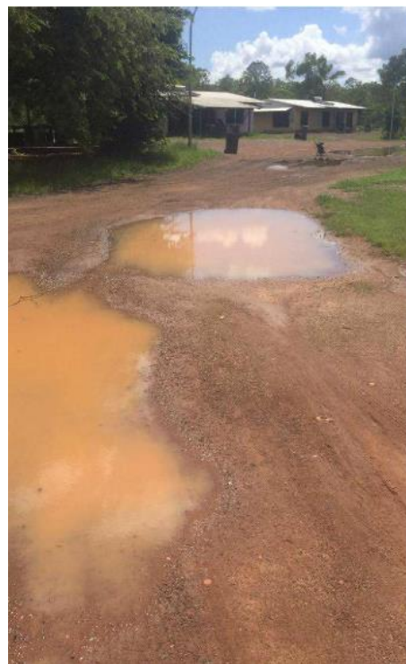
Figure 8 Pavement, condition: very poor
