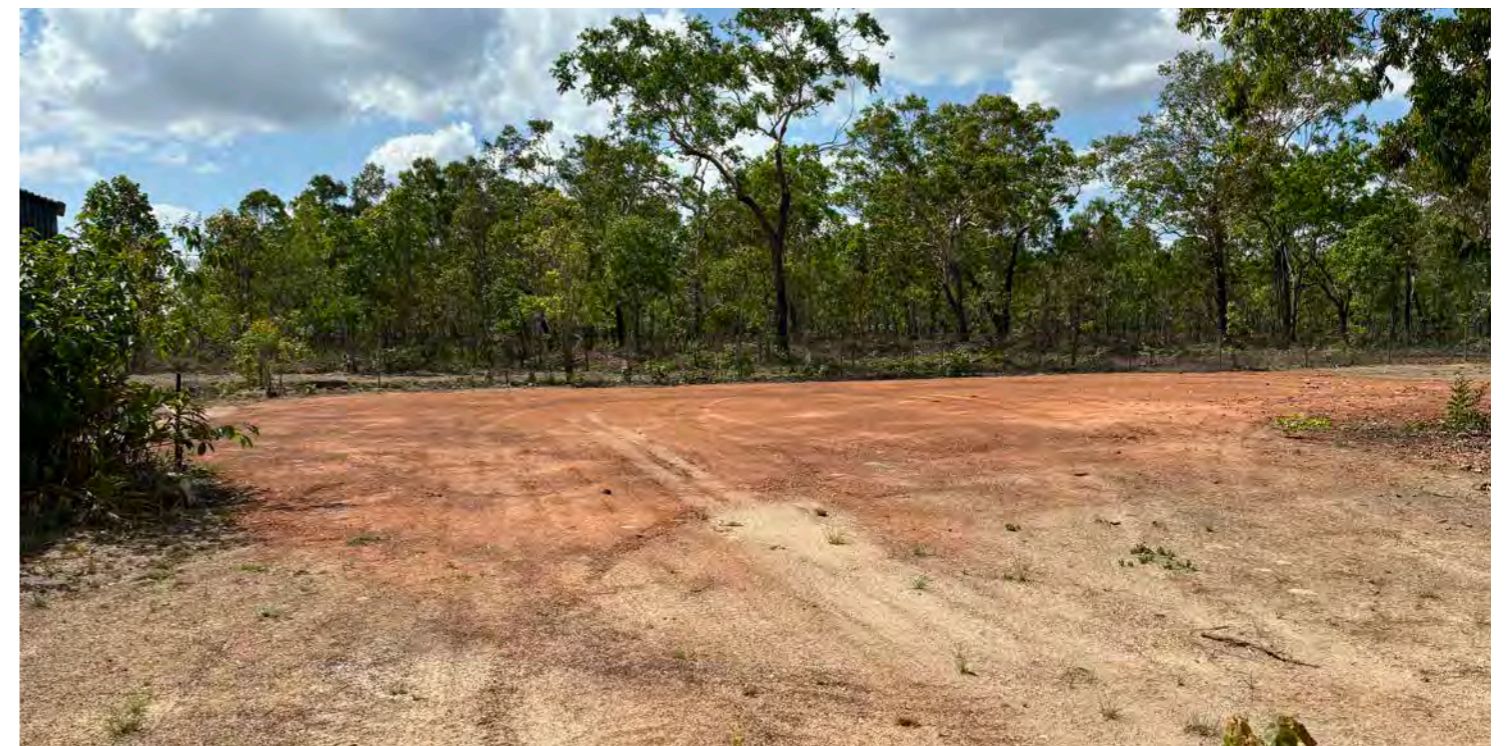
Completed temporary accommodation building pad
