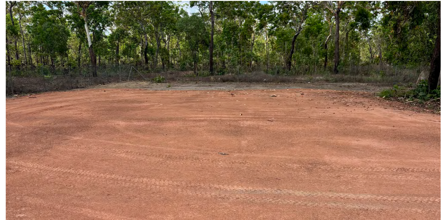
Completed temporary accommodation building pad
