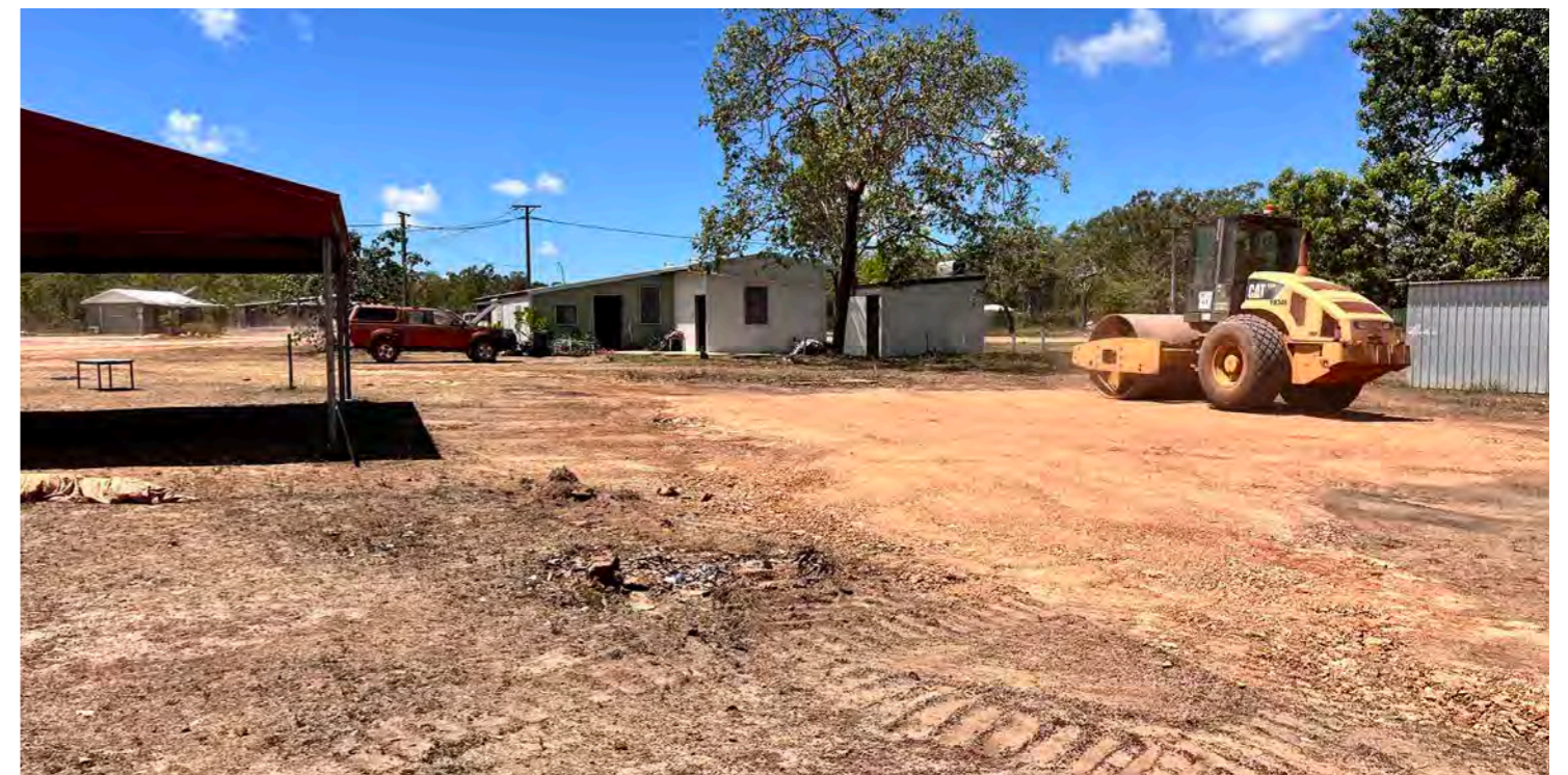
Office demolished for temporary accommodation
