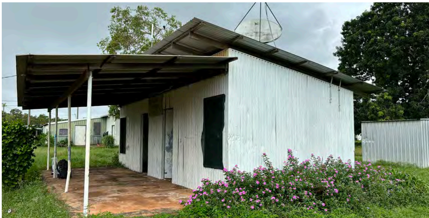
Existing office prior to demolition
