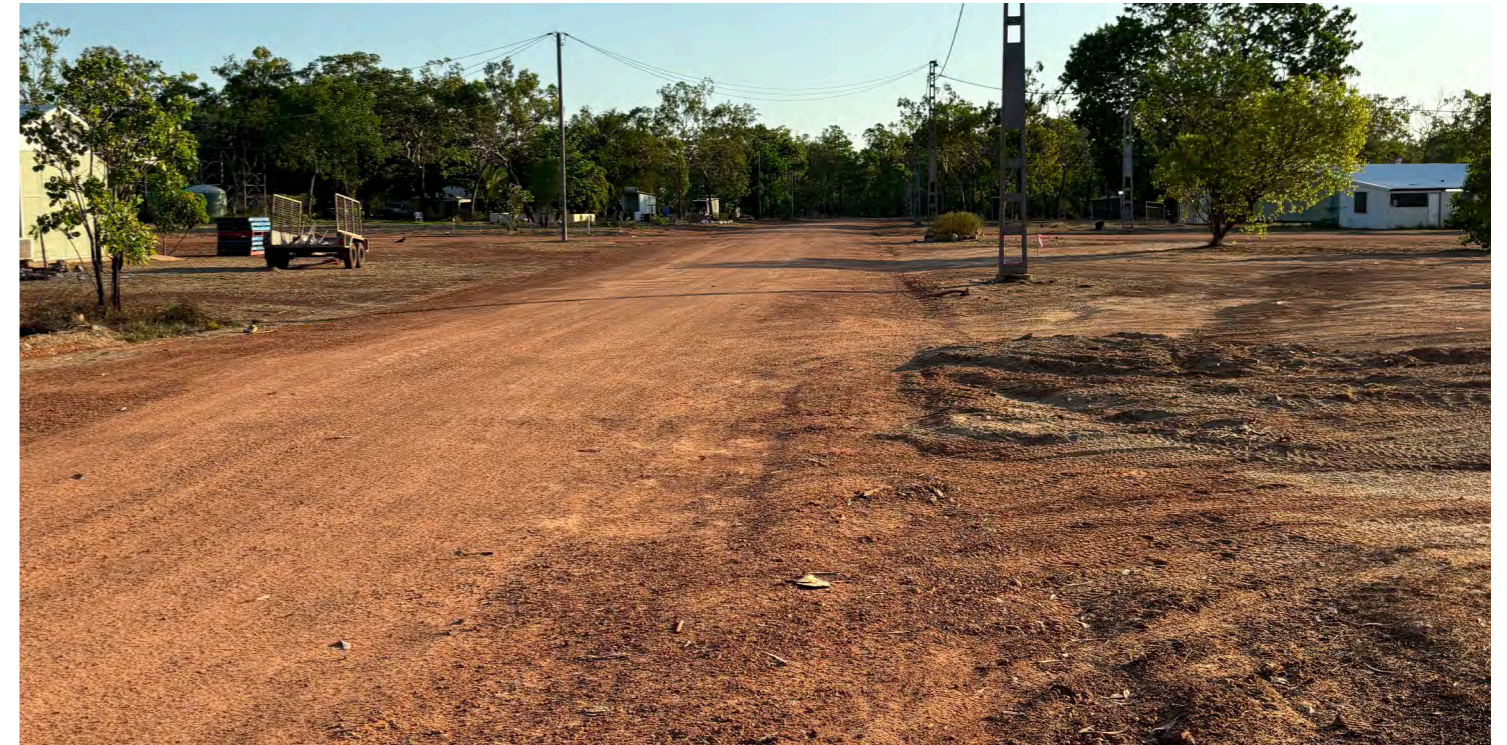
Completed road upgrade, internal road running north/ south
