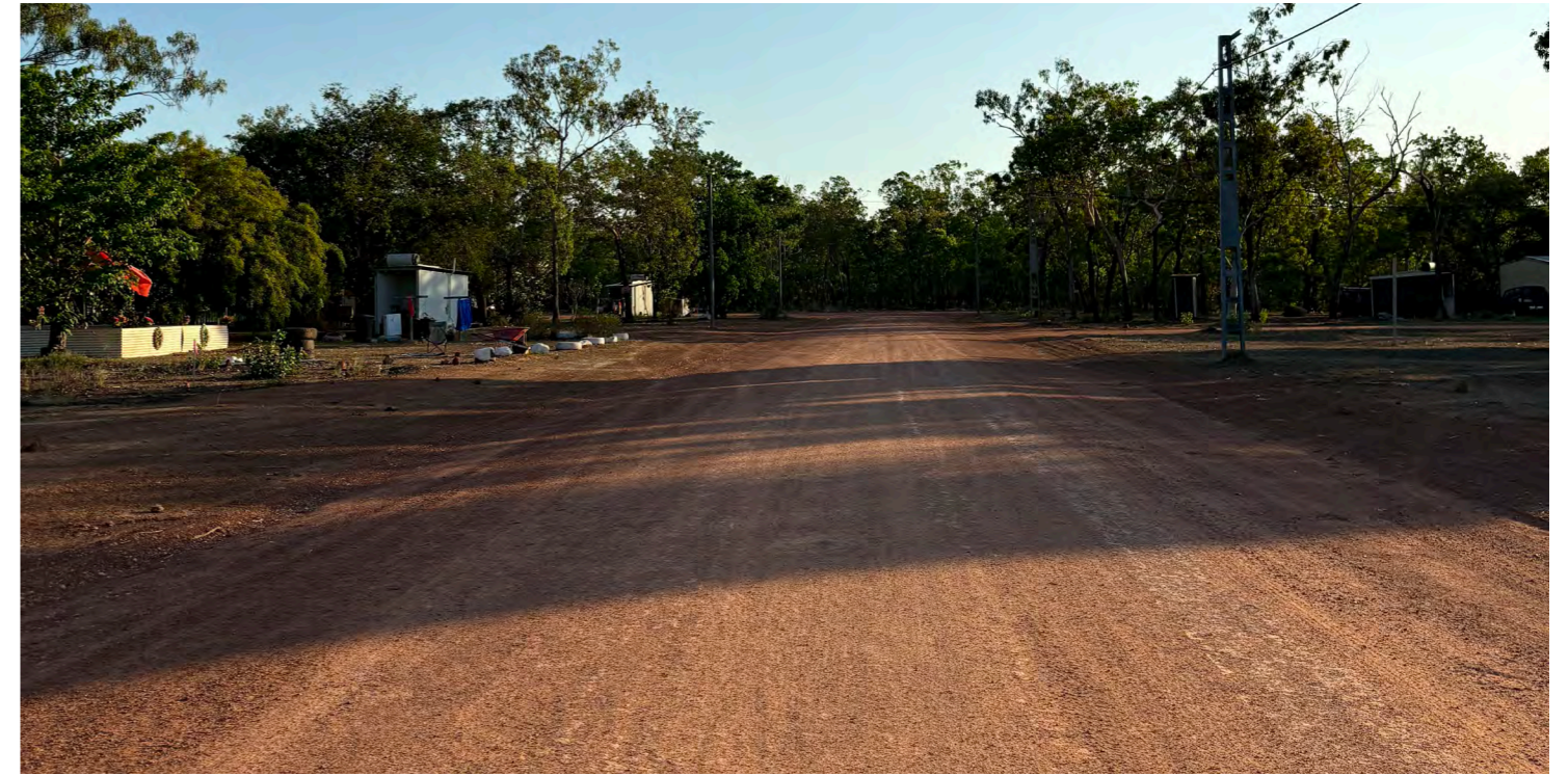
Completed road upgrade to internal road running north/ south
