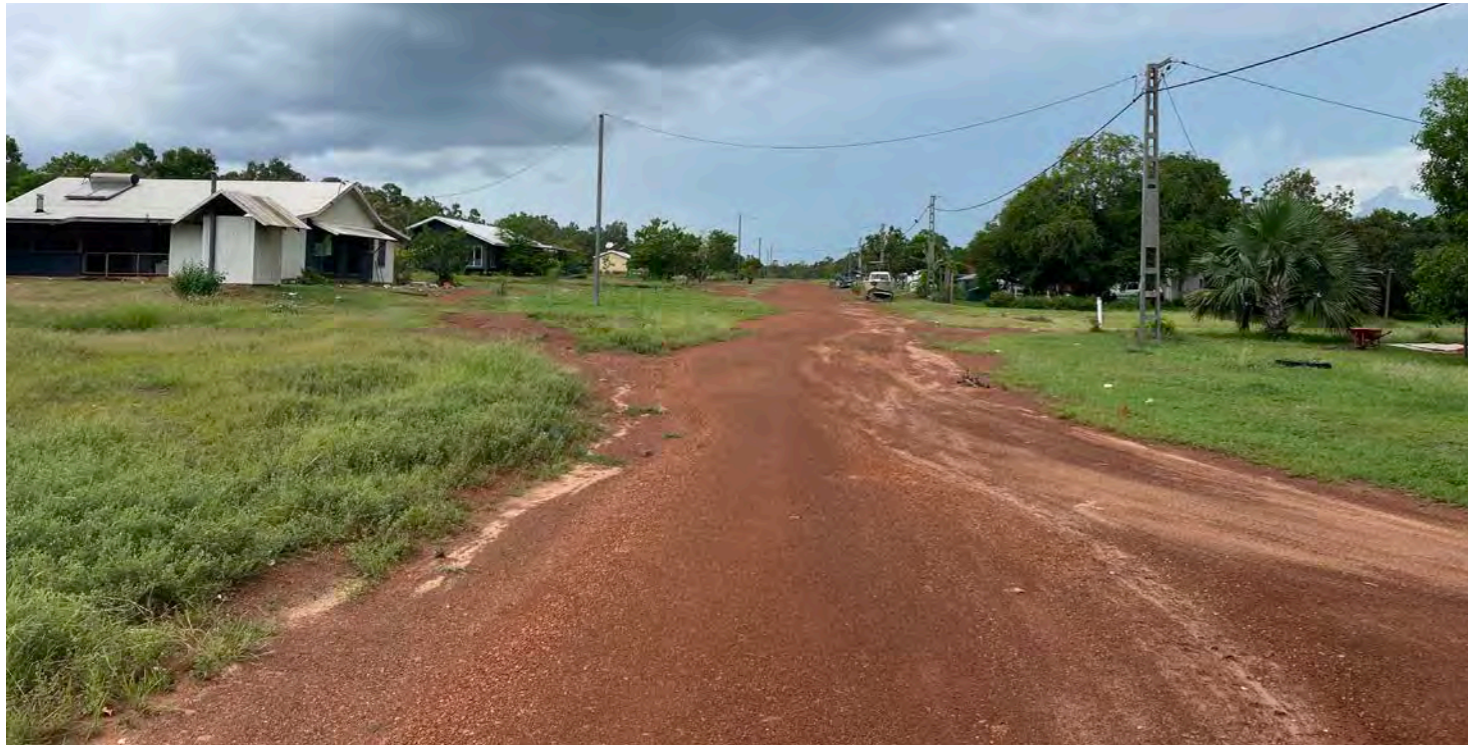
Before photo of internal road running view east/ west
