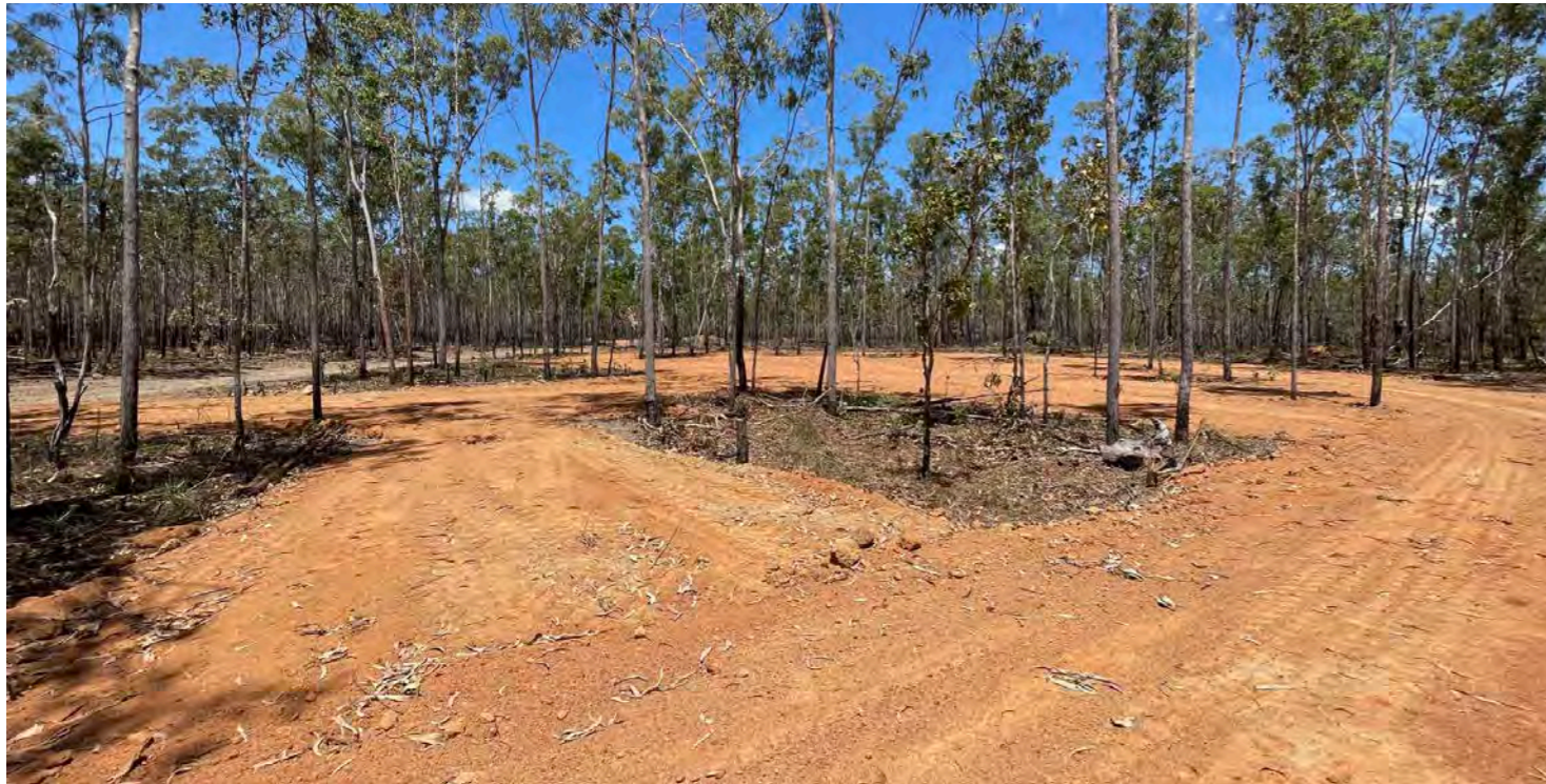
Contractors camp building pad and clearing
