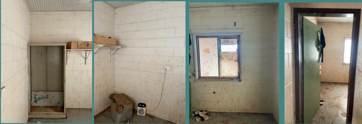
Before Bedrooms works commenced:
