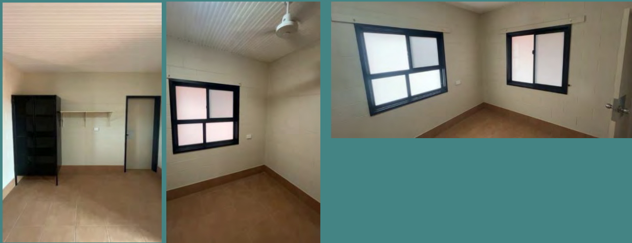
After Bedrooms works completed:
