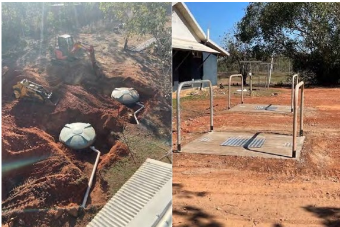
Figure 52. Septic system replacement at Gängan
