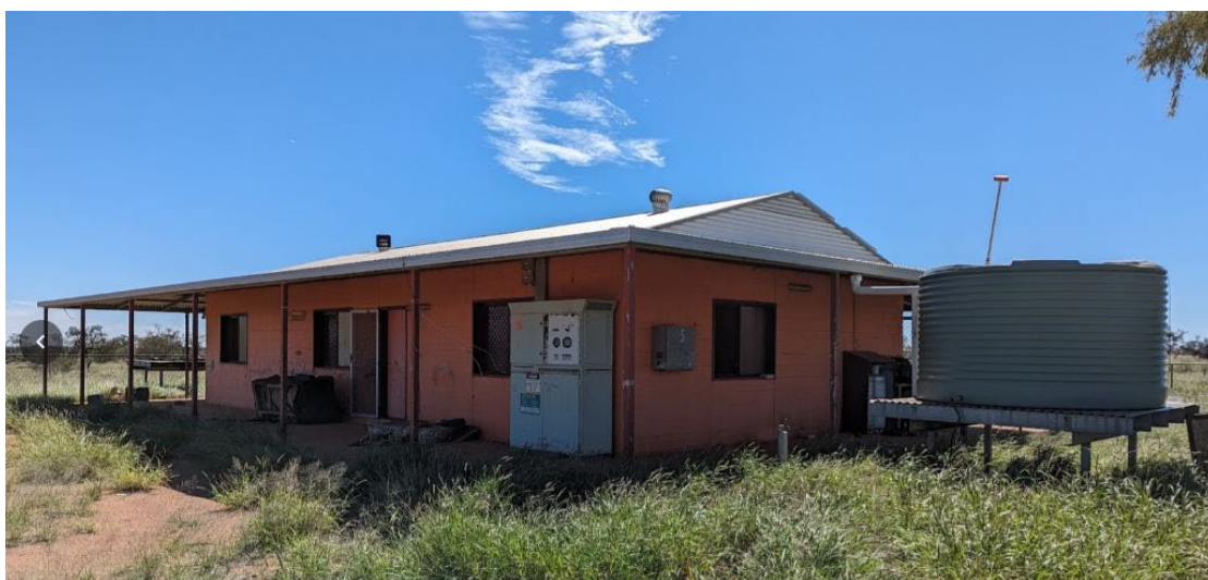
Figure 32. Corkwood Bore house with Bushlight Household RE System
