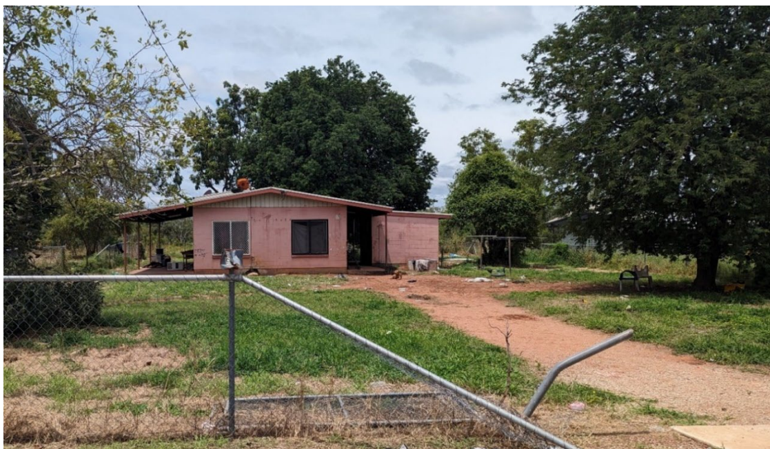
Figure 19. House at Rockhole in March 2024, prior to refurbishment
