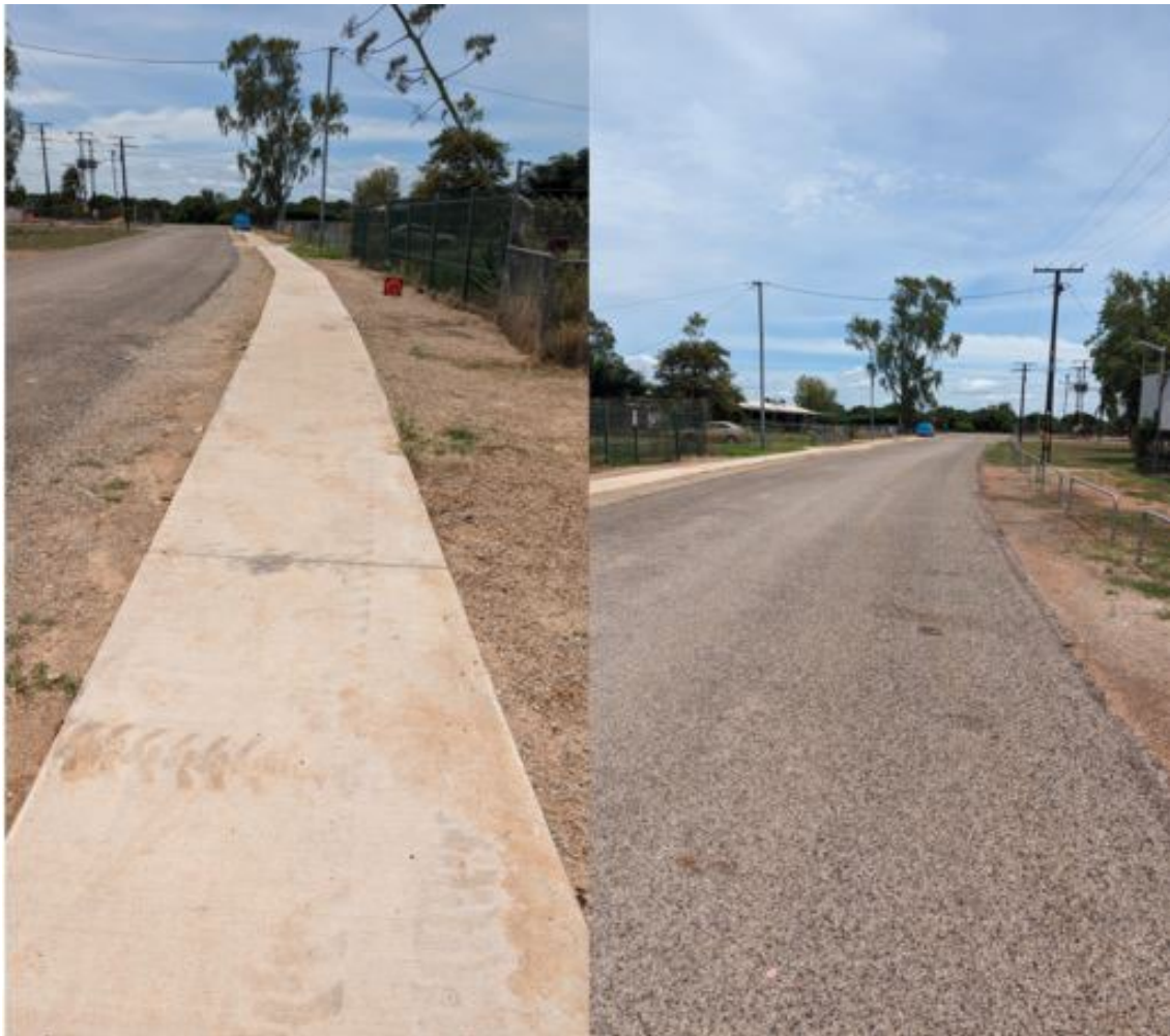
Figure 23. New footpath (left), improved road and bollards around oval area (right)
