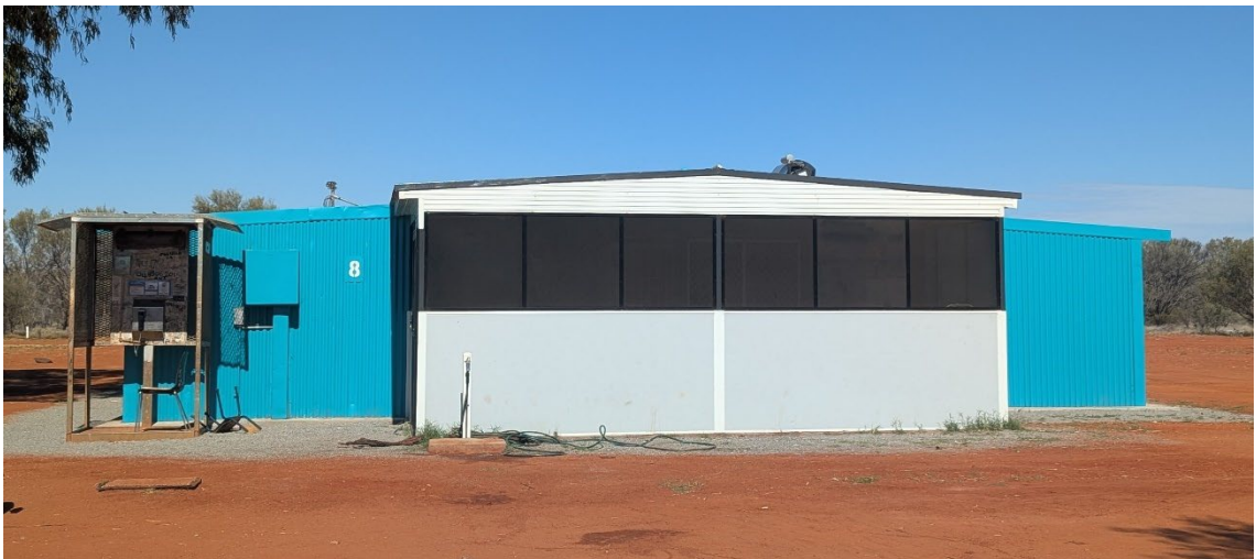
Figure 45. Renovated dwelling at Burt Creek, July 2025
