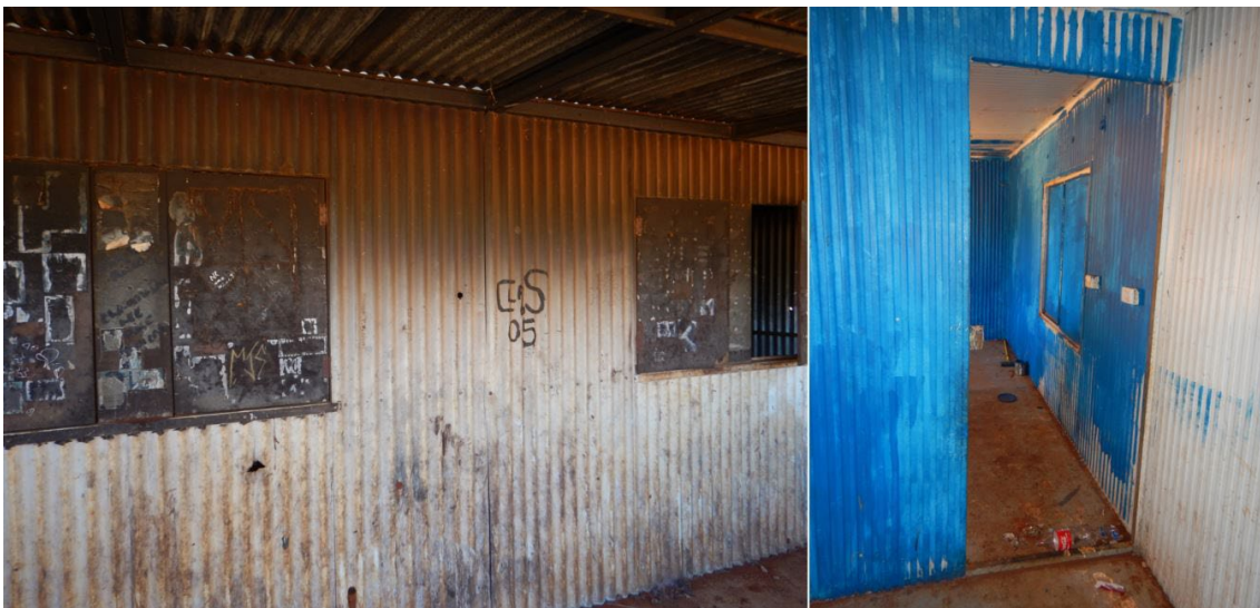
Figure 40. Burt Creek tin dwelling prior to HEA upgrades
