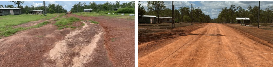
Figure 53. East-west road before and during civil works
