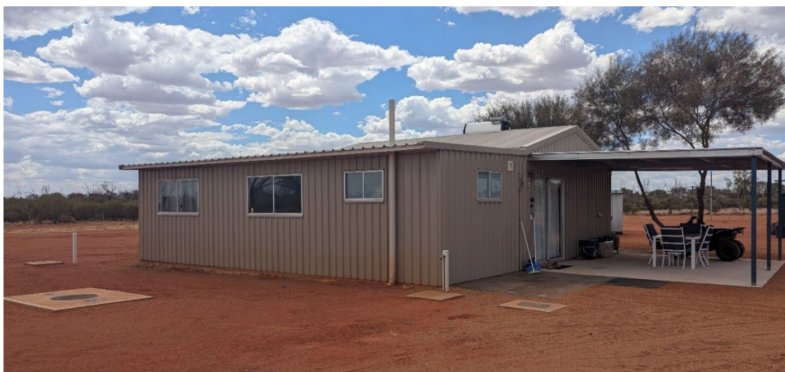
Figure 37. Completed renovation at Anpanaye
