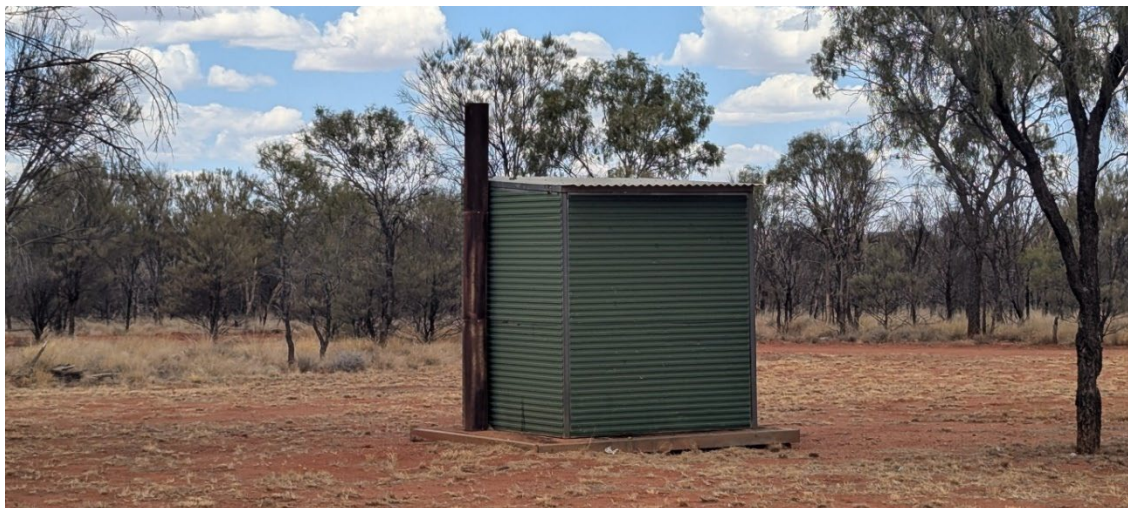
Figure 58. Ventilation improved pit (VIP) toilet in Central Australian homeland
