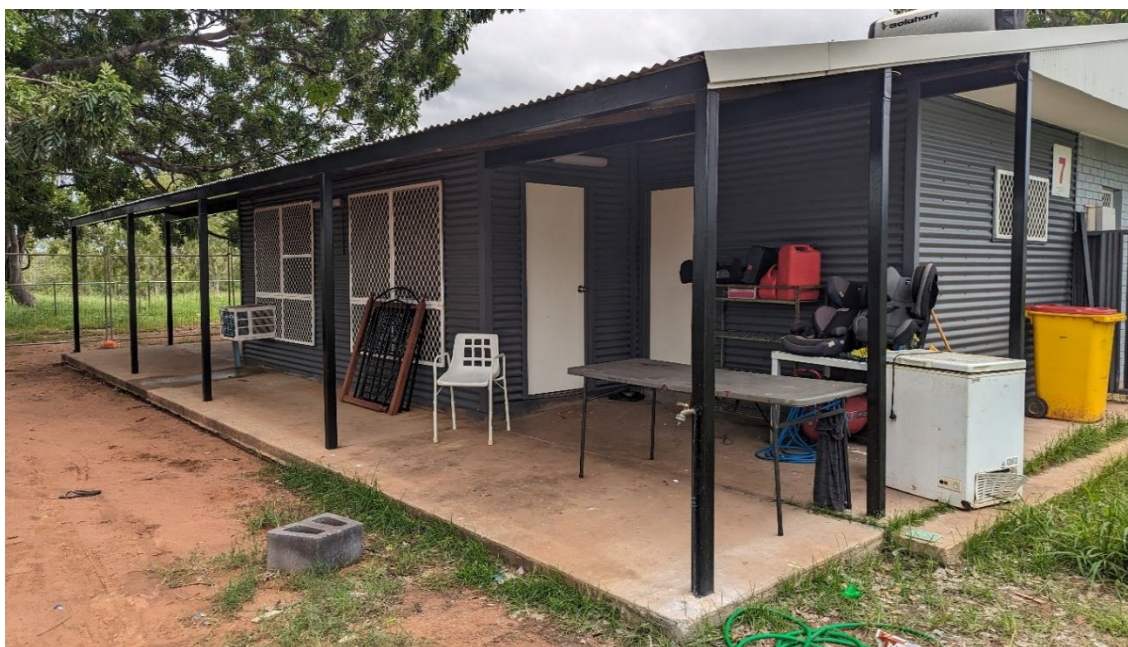
Figure 25. Refurbished house, additional bedroom to come at back left
