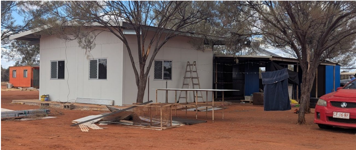
Figure 44. In-process extension at Burt Creek, March 2025
