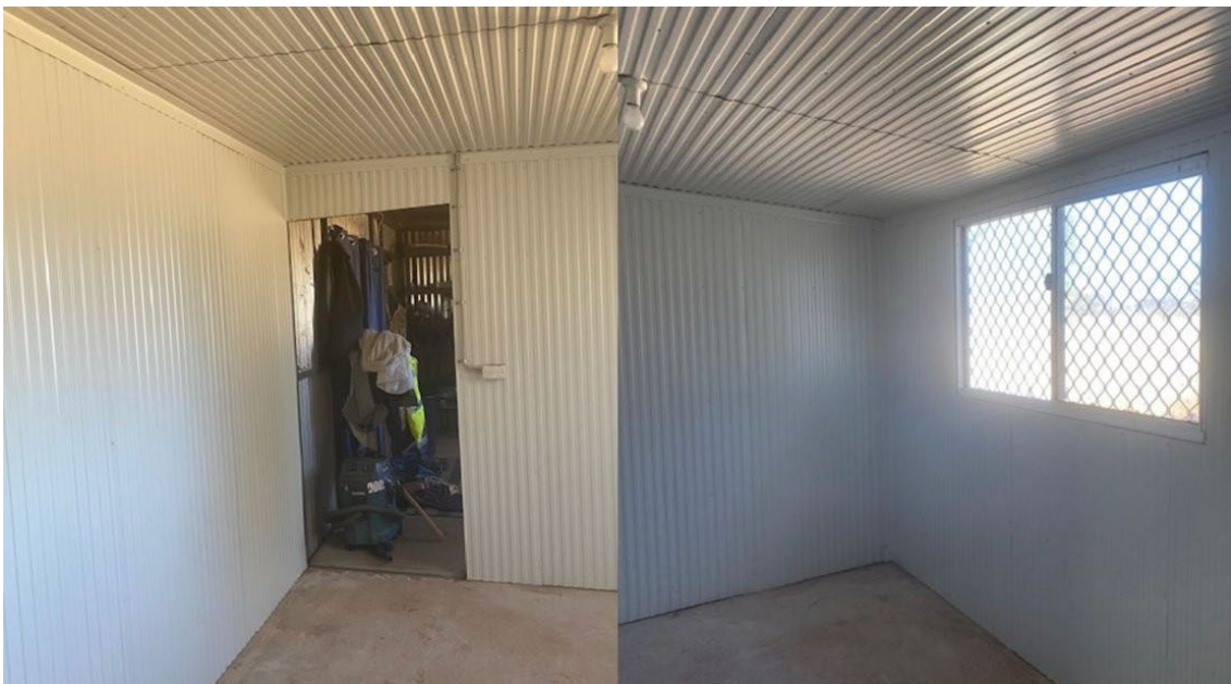
Figure 41. Burt Creek tin shed dwelling after Homelands Extras Allowance upgrades
