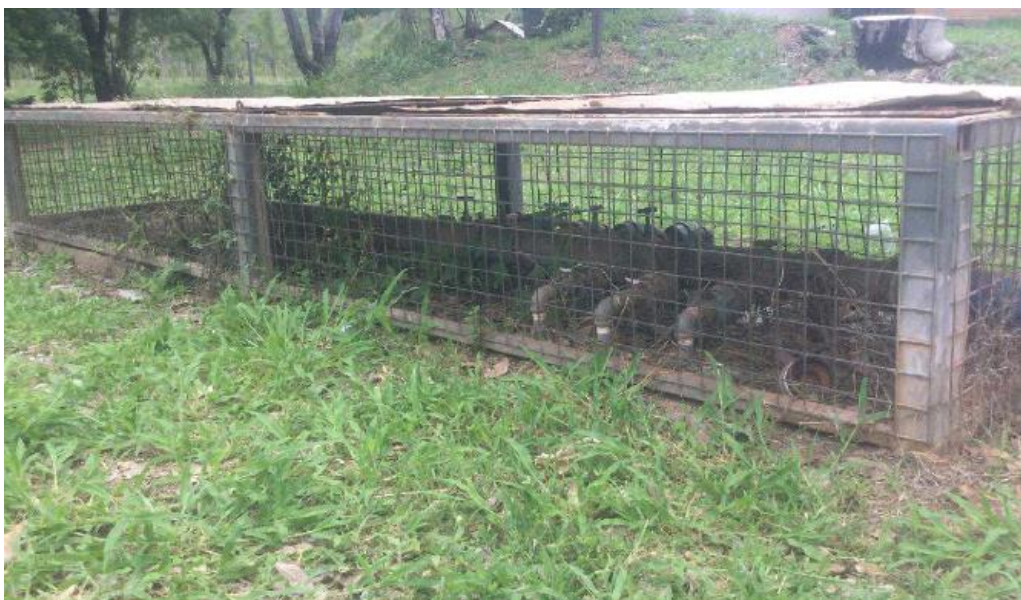
Figure 2 Residential lot water meters, condition: poor
