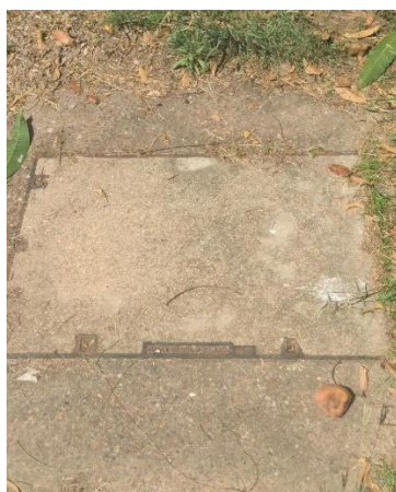
Figure 2 Manhole, condition: very good
