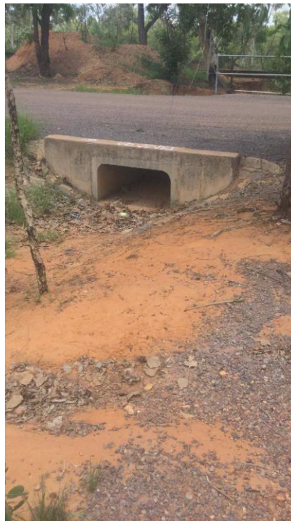
Figure 8 Headwall and culvert, condition: very good
