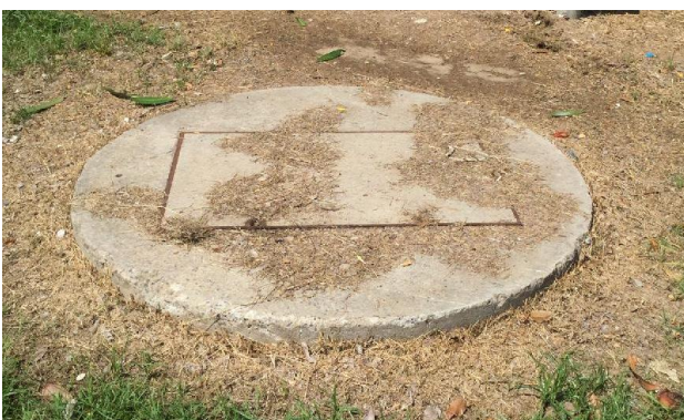
Figure 1 Manhole, condition: good
