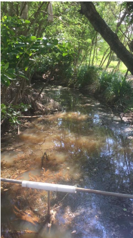
Figure 10 Drain with ponding
