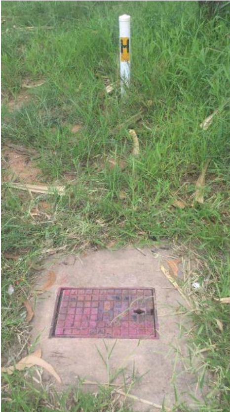
Figure 3 Fire hydrant, condition: good
