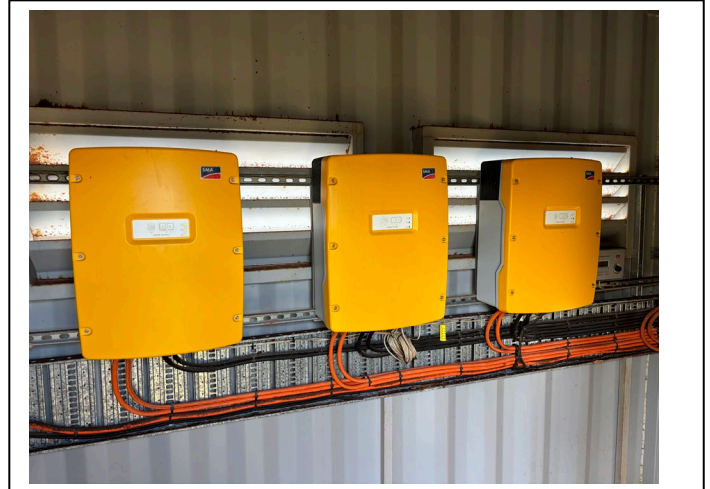
Existing SMA inverter / chargers
