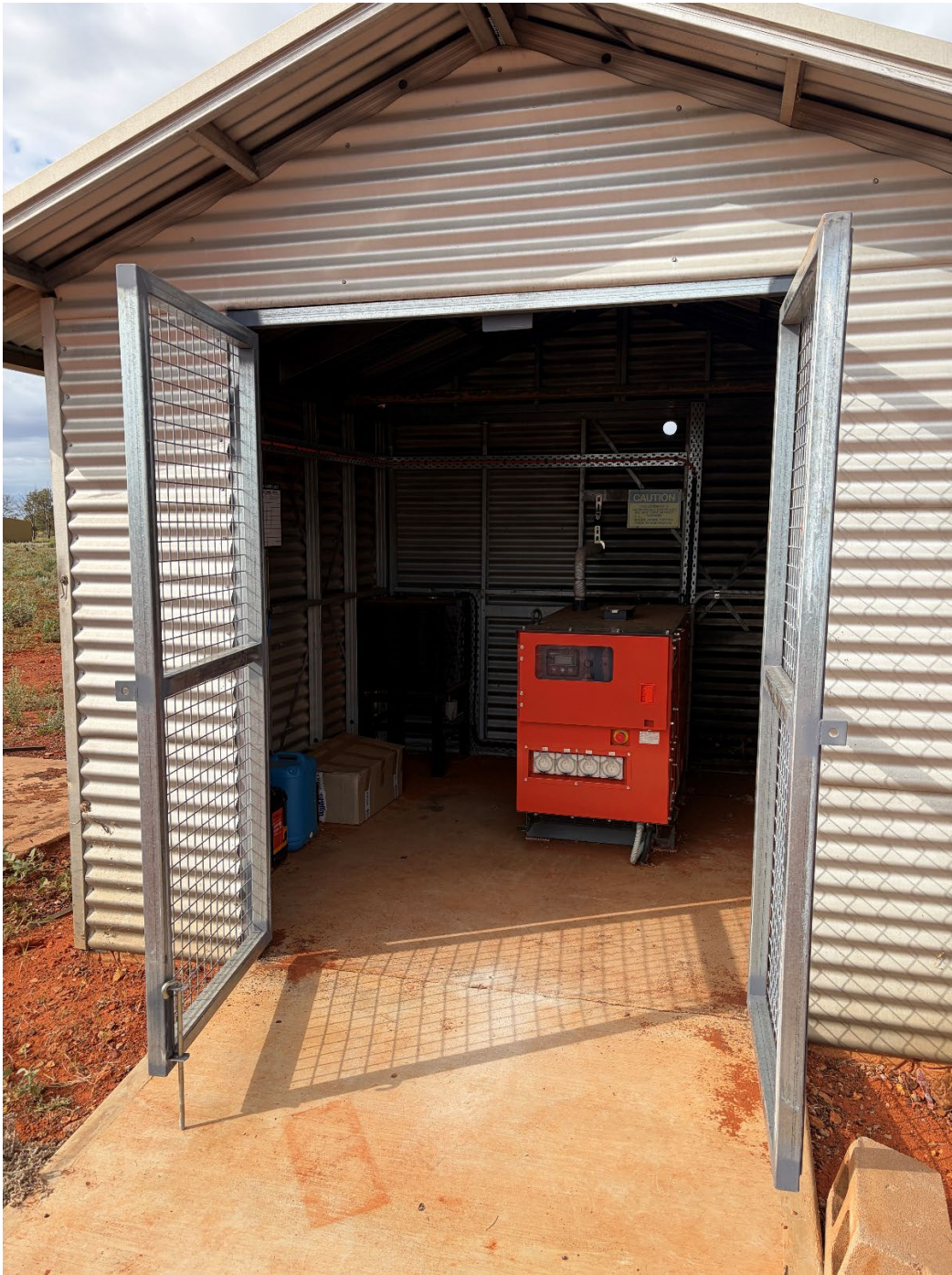
Replace Gate to Genset Shed
