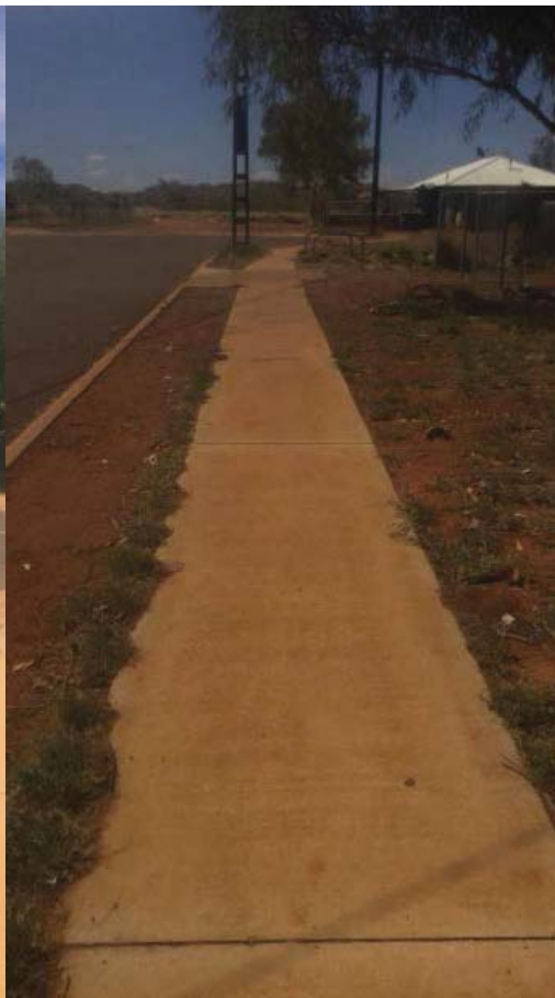
Figure 8 Footpath, condition: good
