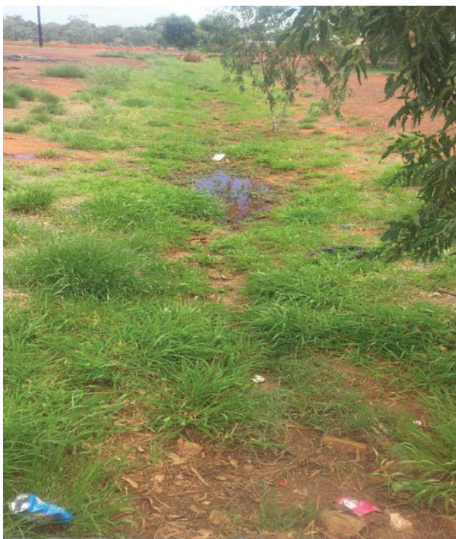
Figure 13 Swale, condition: good . Ponding due to hose left on nearby.
