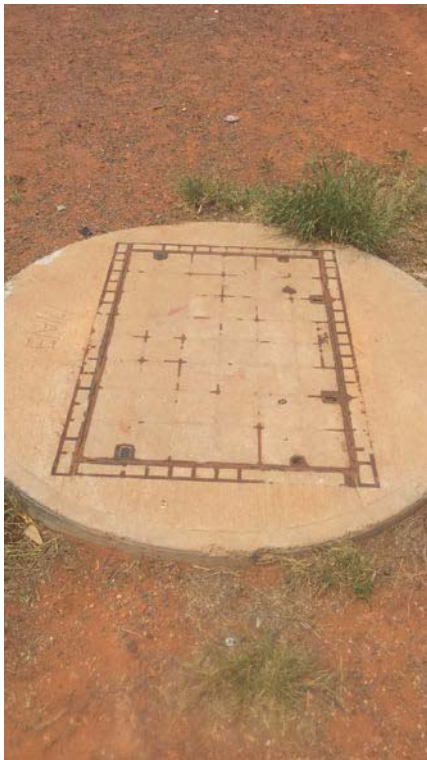
Figure 1 Sewer manhole, condition: good
