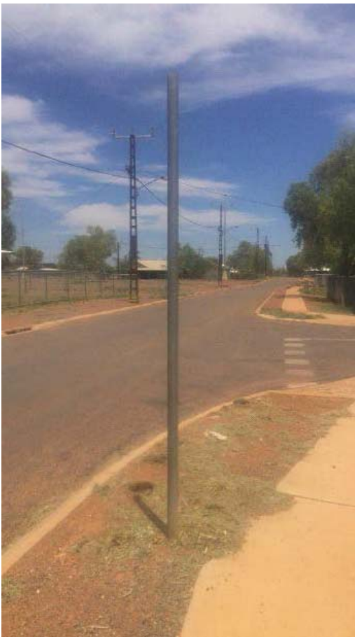
Figure 7 Sign, condition: very poor
