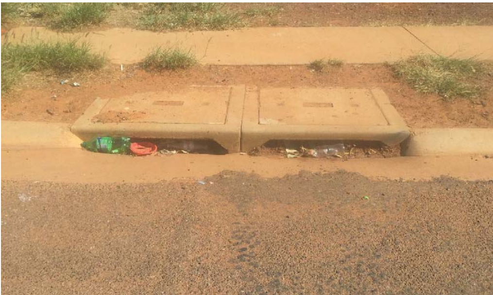
Figure 12 Two bay side entry pit, condition: good
