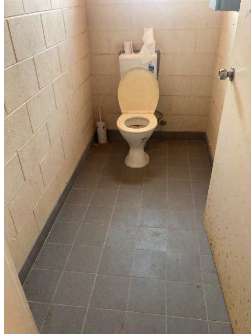
Tiling to WC:
