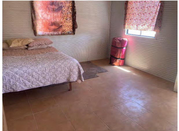
Tiling to extension floor:
