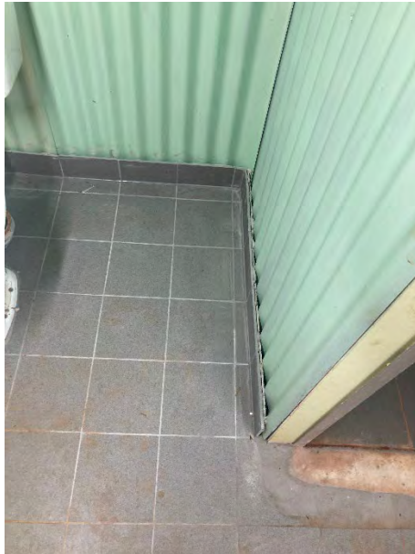
Tiling to bathroom:
