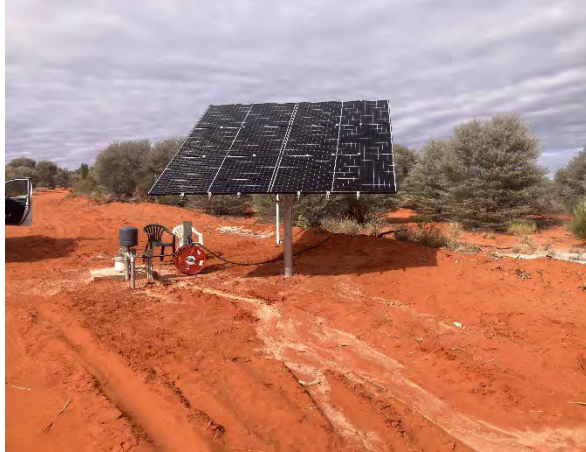
Solar fixed array installed:
