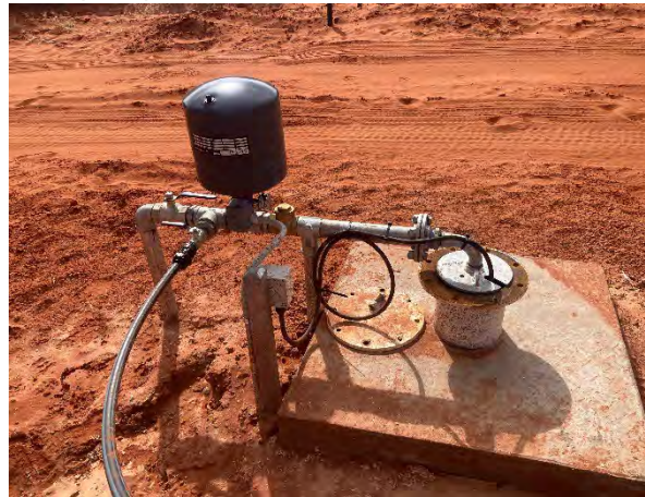
Bore pump installed:
