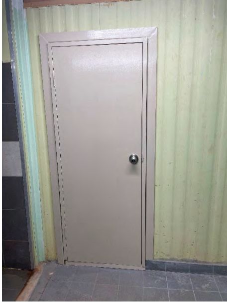
Door from bathroom into demountable:
