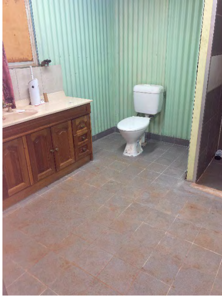
Tiling to bathroom:
