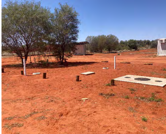
New septic system:
