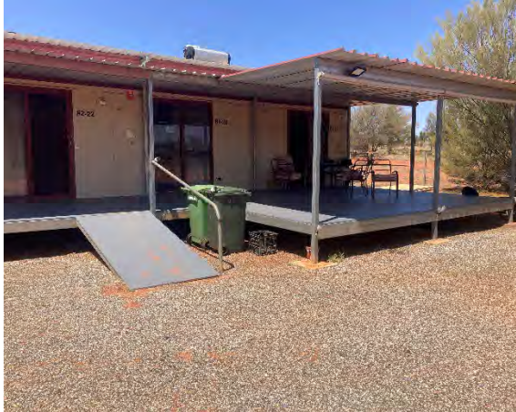
Deck sheets re-laid and painted
