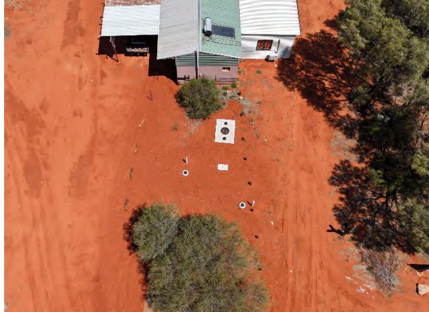
New septic system:
