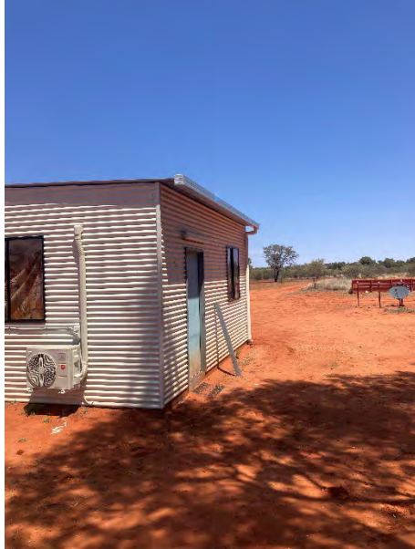
Split system and guttering installed:
