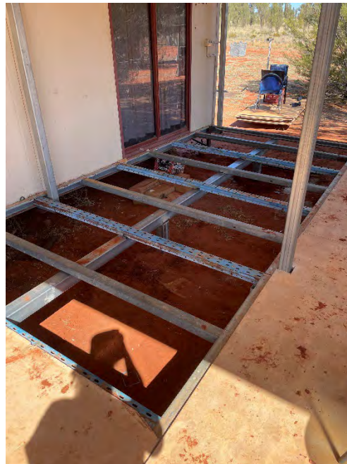
Deck bearer installed:
