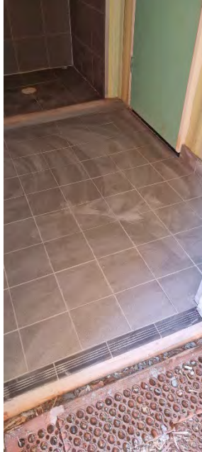
Tiling to bathroom:
