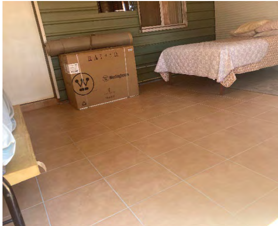
Tiling to extension floor:
