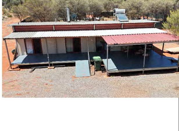
Deck sheets re-laid and painted
