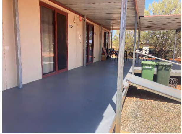
Deck sheets re-laid and painted
