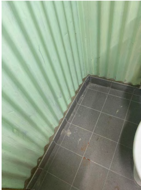
Tiling to bathroom:
