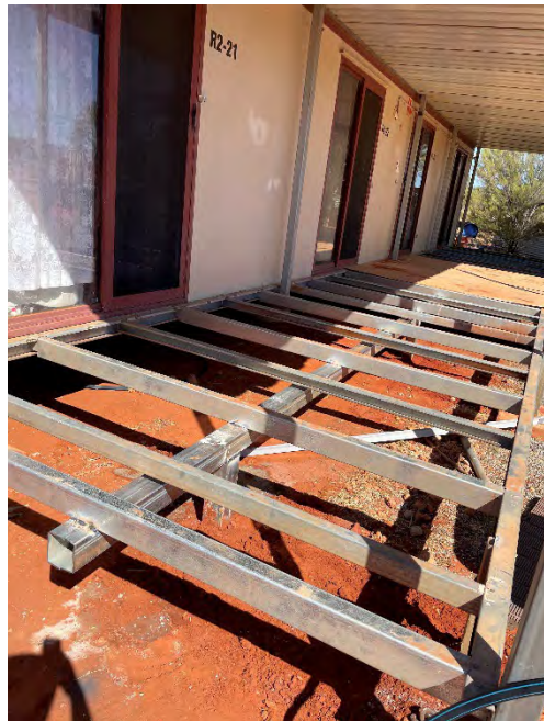
Deck bearer installed:
