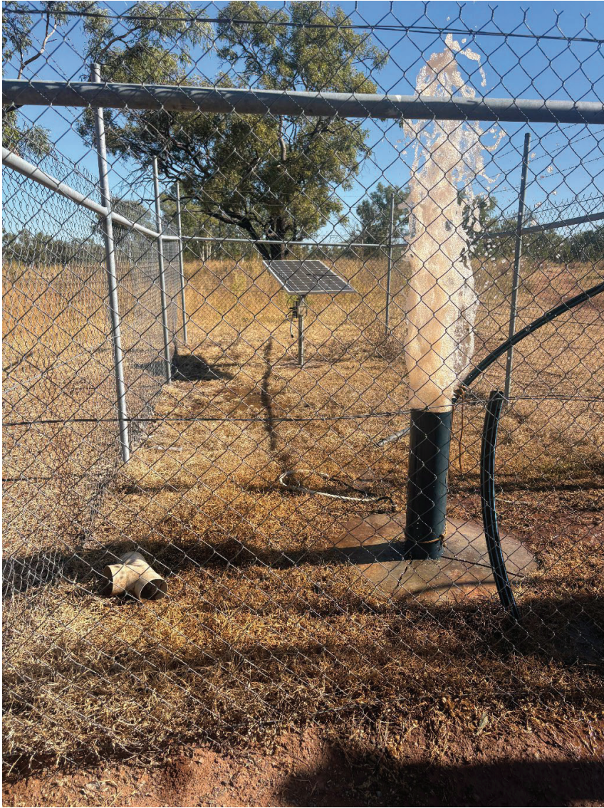
Bore rehabilitation at 39119 Fitzroy Station
