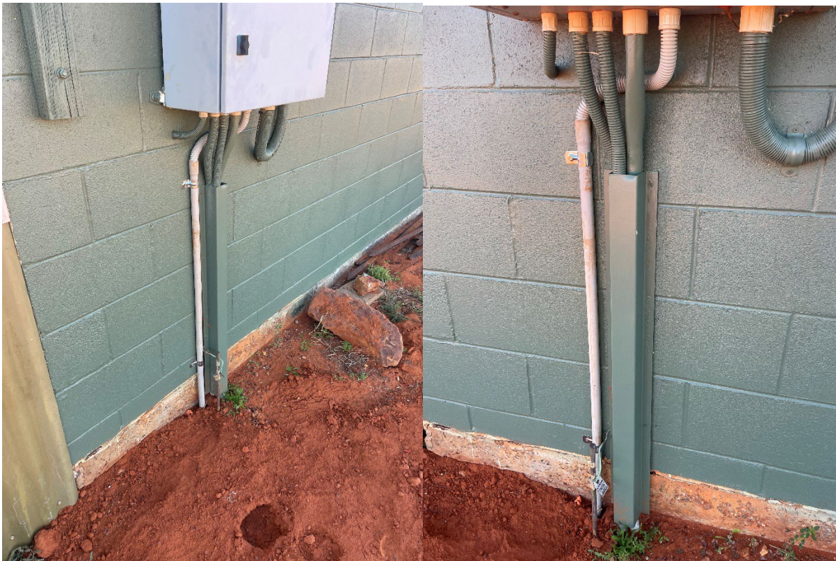
Electrical Connection run new feed to H4
