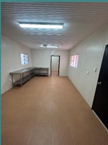
After works completed:
