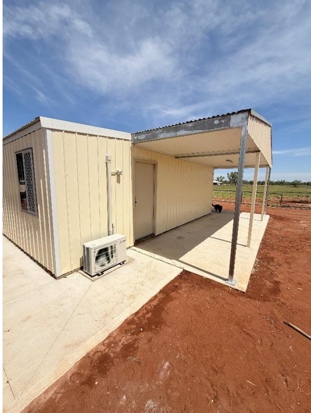
Front door and veranda:
