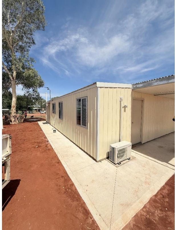
Concrete path and rear door:
