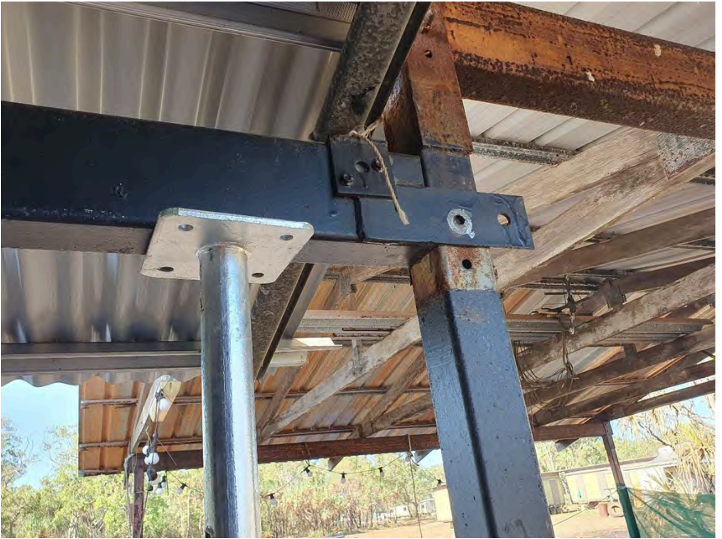
Rear verandah roof raised for better alignment
