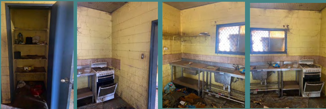
Before works commenced:
