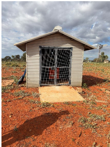
Replace Gate to Genset Shed
