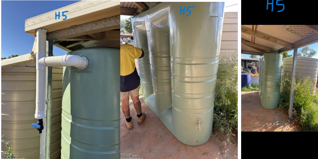
Installed rainwater tank on house 4
