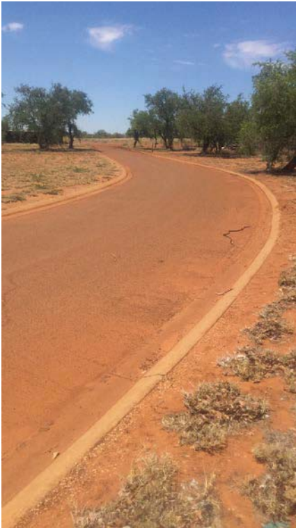
Figure 8 Bindjaeni Court, condition: good
