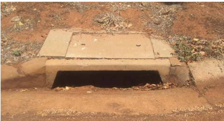
Figure 13 One bay side entry pit, condition: good
