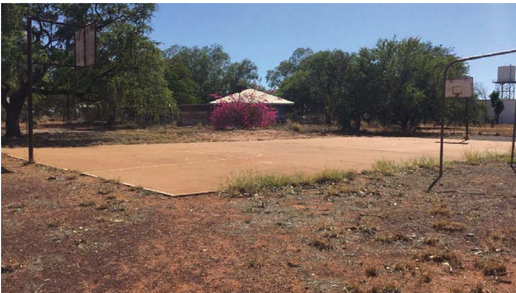
Figure 14 Basketball court, condition: poor
