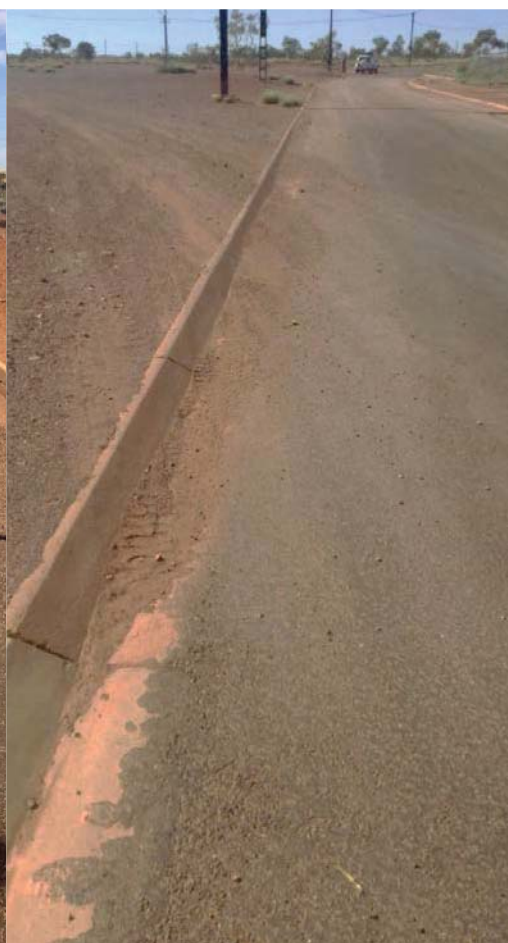
Figure 10 Gurungu Street, condition: good
