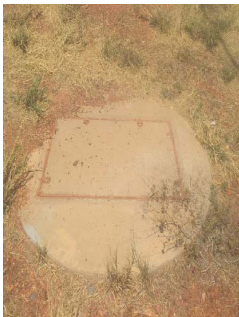
Figure 1 Sewer manhole, condition: good
