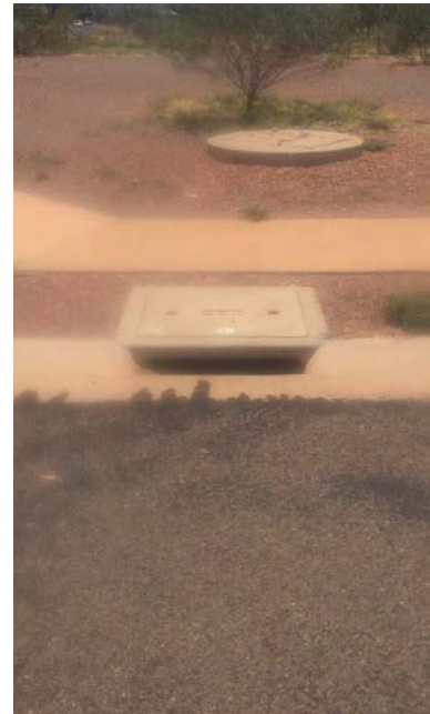
Figure 12 One bay side entry pit, condition: very good
