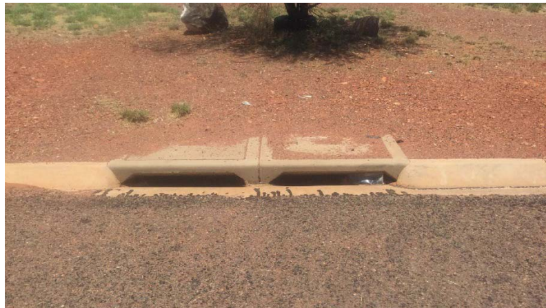
Figure 13 Two bay side entry pit, condition: very good
