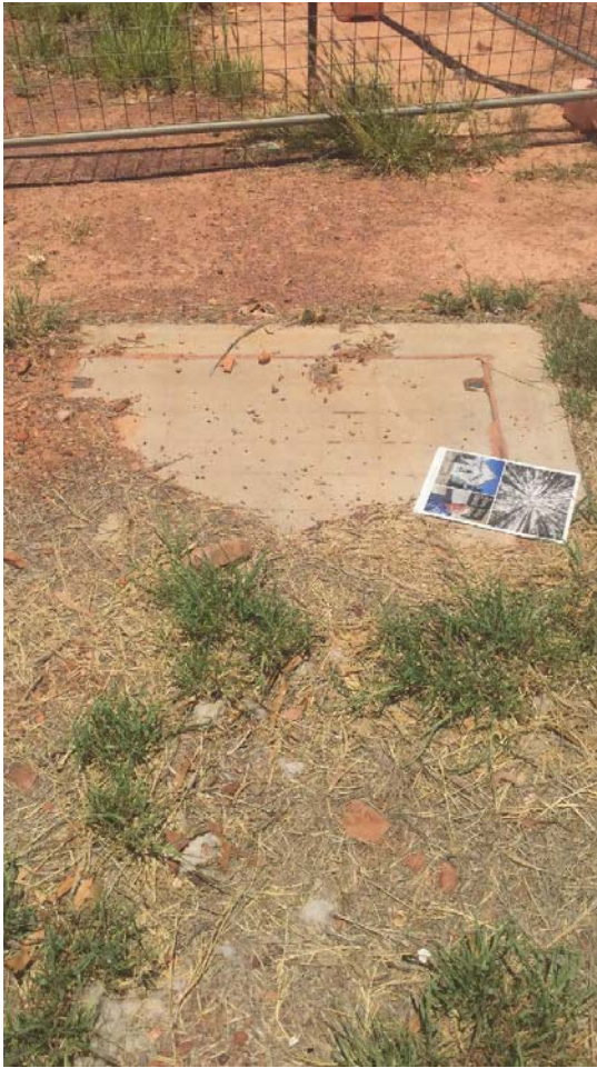
Figure 1 Sewer manhole, condition: good
