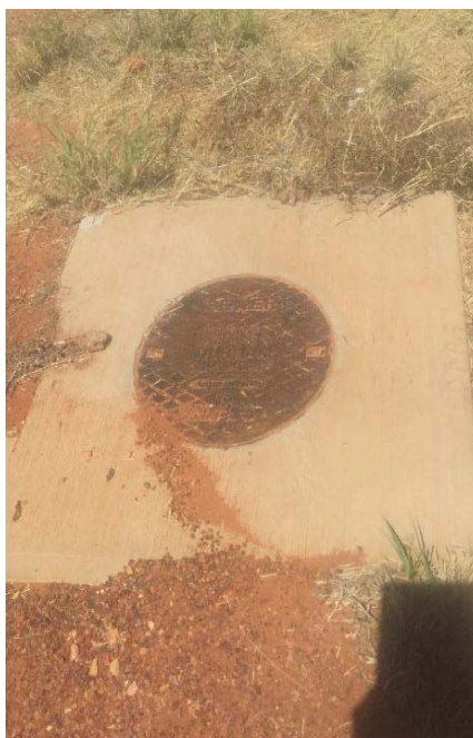
Figure 2 Sewer manhole, condition: very good
