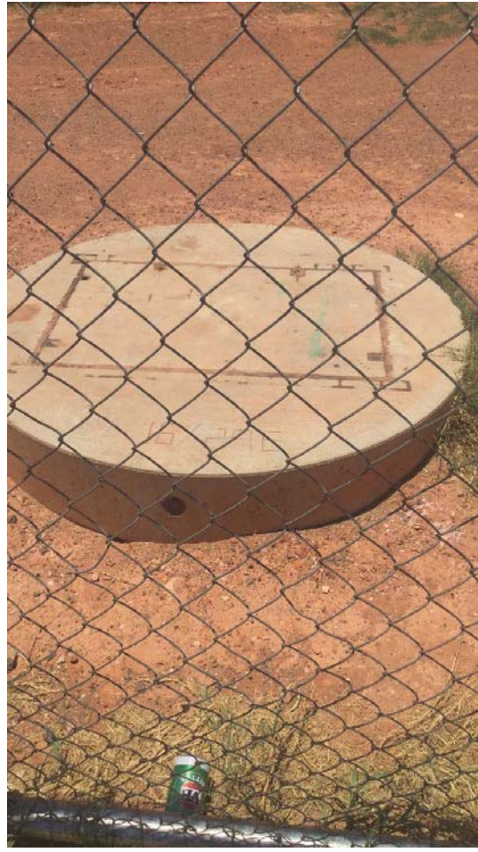
Figure 2 Sewer manhole, condition: very good
