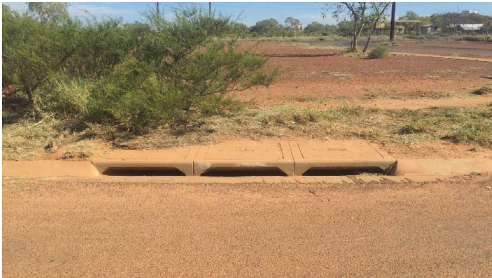
Figure 13 Three bay side entry pit, condition: very good
