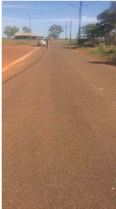
Figure 10 Road 238_4, condition: good
