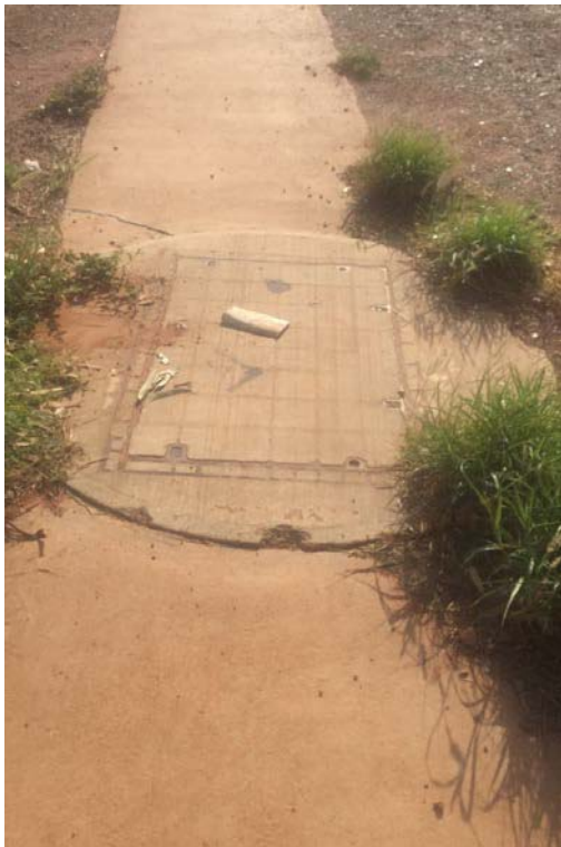
Figure 1 Sewer manhole, condition: good
