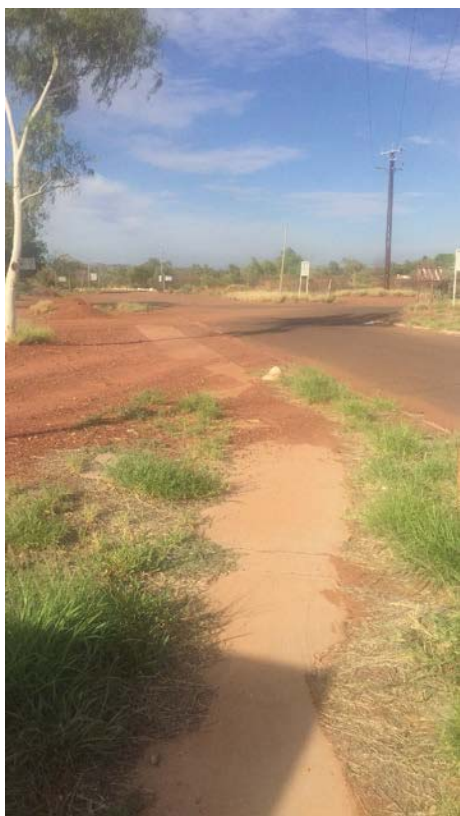
Figure 6 Footpath, condition: good
