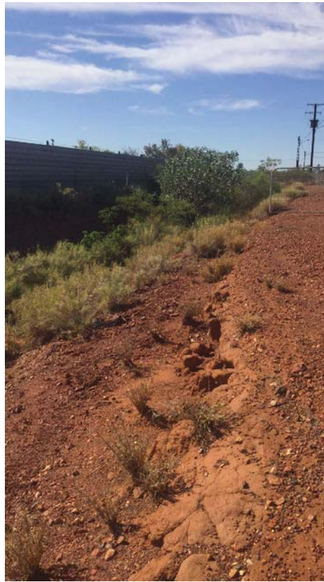
Figure 12 Swale, condition: good
