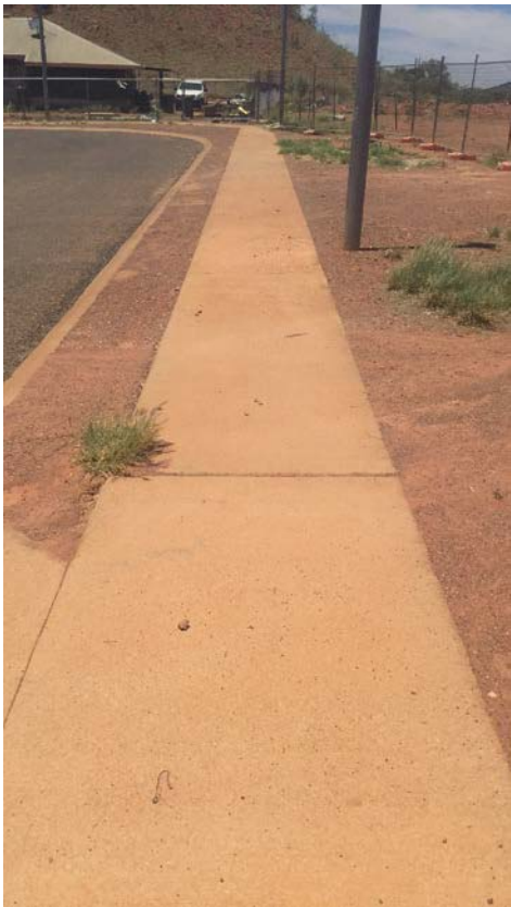
Figure 7 Footpath, condition: good
