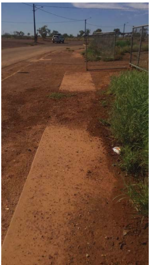
Figure 7 Footpath, condition: good
