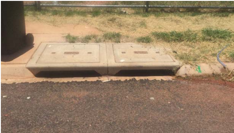
Figure 11 Two bay side entry pit, condition: very good
