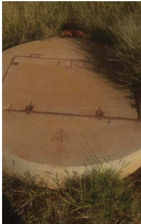
Figure 2 Sewer manhole, condition: very good
