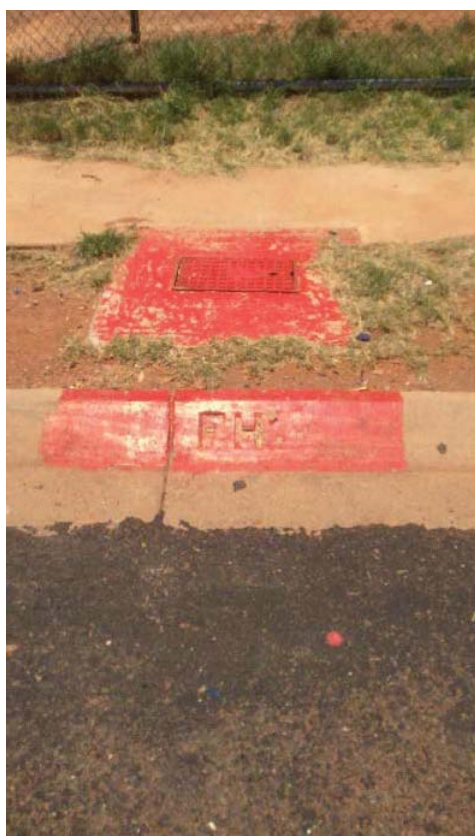
Figure 4 Fire hydrant, condition: very good
