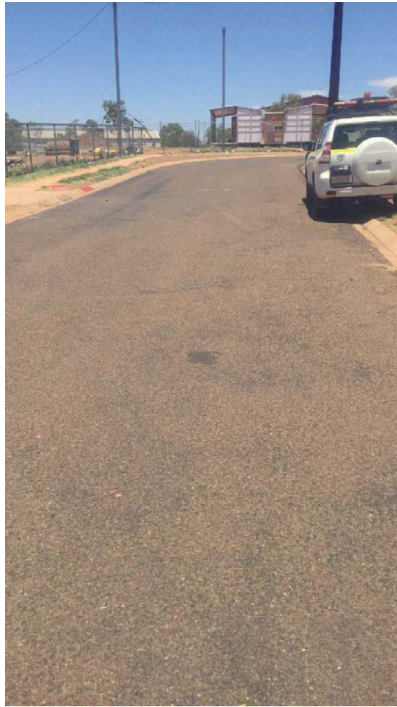
Figure 10 Road 215_1, condition: good
