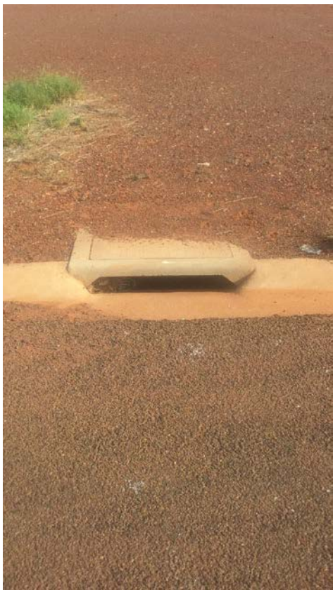
Figure 11 One bay side entry pit, condition: good
