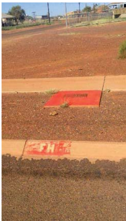
Figure 5 Fire hydrant, condition: good
