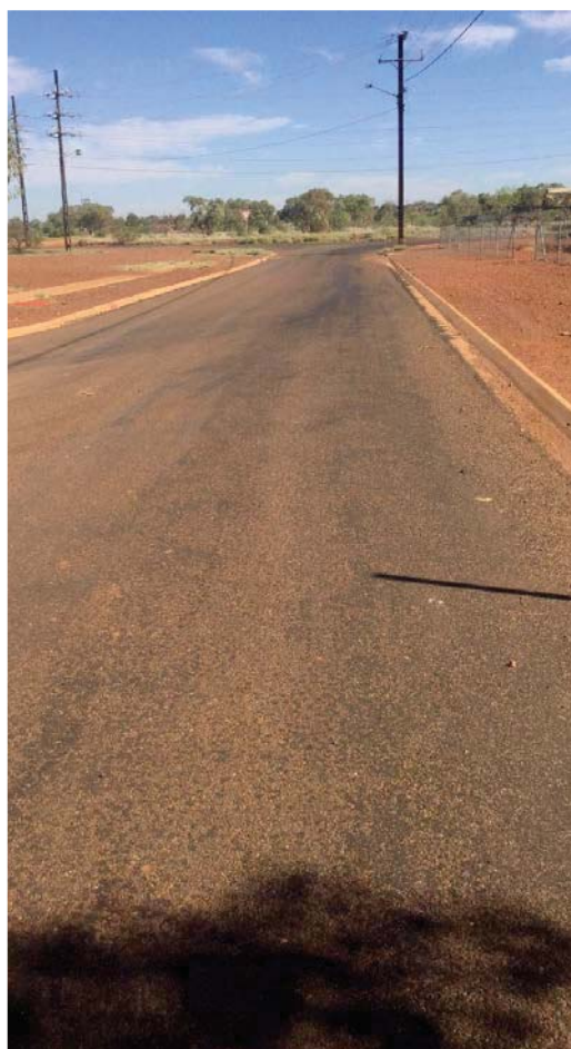
Figure 9 Gurungu Street, condition: good
