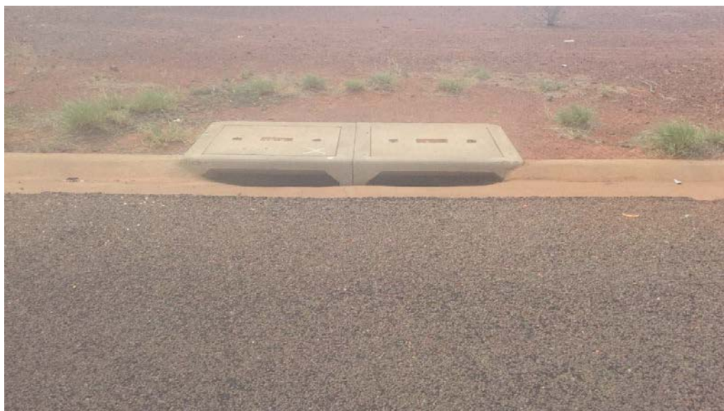
Figure 12 Two bay side entry pit, condition: very good
