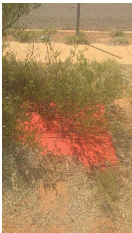
Figure 4 Fire hydrant, condition: good
