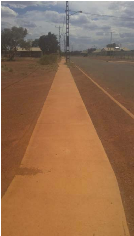
Figure 7 Footpath, condition: very good
