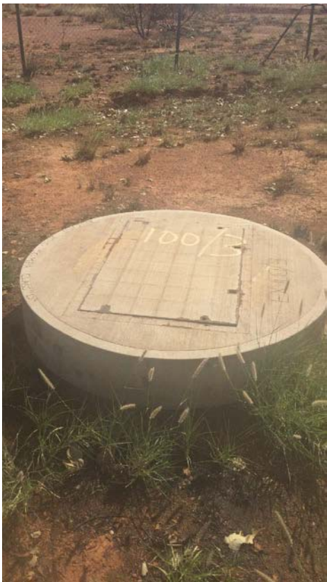
Figure 1 Sewer manhole, condition: very good
