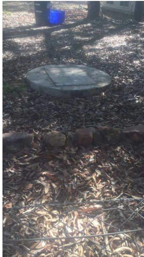
Figure 2 Sewer manhole, condition: good
