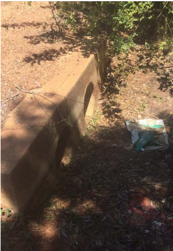
Figure 14 Twin RCP culvert and headwall, condition: good
