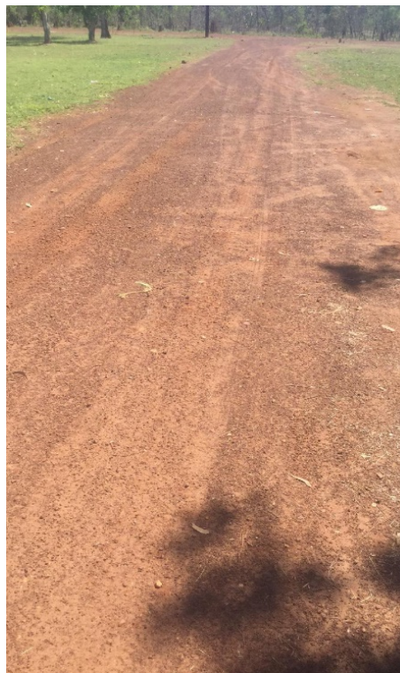
Figure 13 Pavement, condition: good
