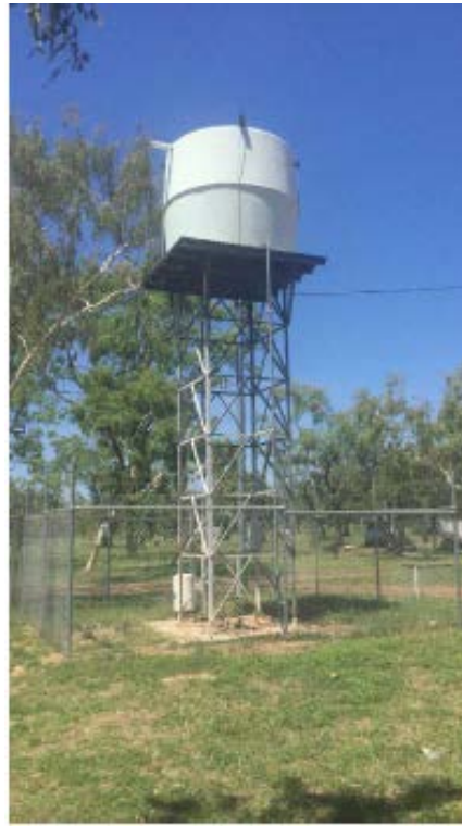
Figure 7 Water tank, condition: good
