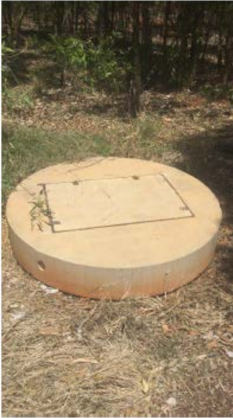
Figure 1 Sewer manhole, very good condition
