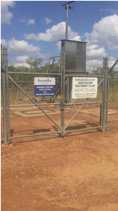
Figure 1 Sewage pump station, condition: good
