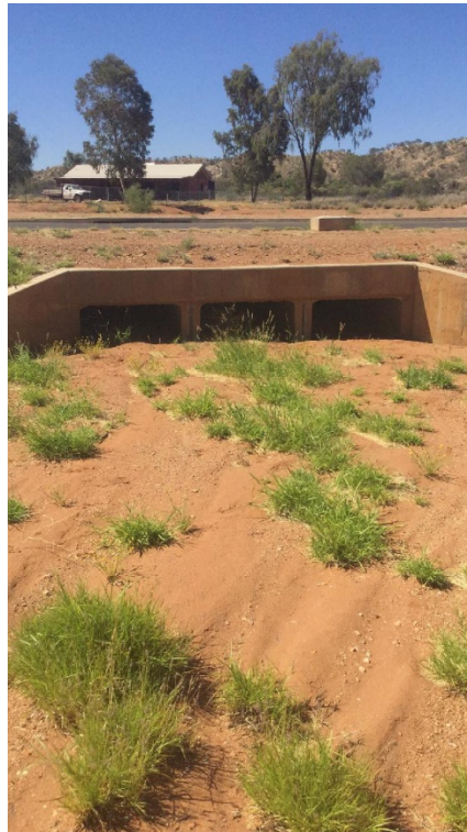
Figure 16 Culver and headwall, condition: very good
