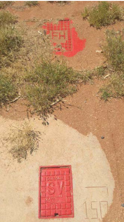
Figure 5 Fire hydrant, condition: good
