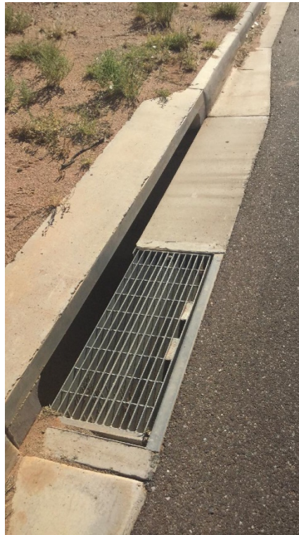
Figure 14 Side entry pit, condition: excellent
