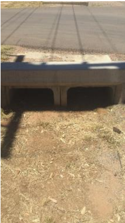
Figure 12 Culvert (upstream), condition: good
