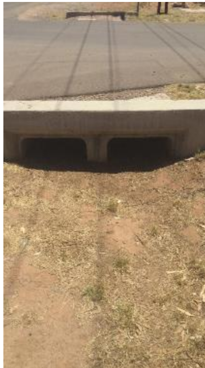
Figure 13 Culvert (downstream), condition: good
