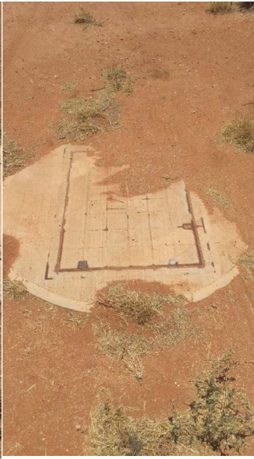
Figure 2 Sewer manhole, condition: very good
