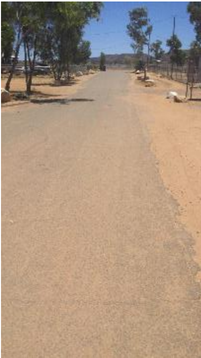
Figure 10 Pavement, condition: good
