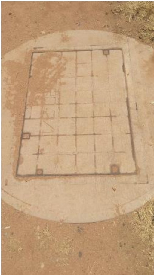
Figure 2 Sewer manhole, condition: very good
