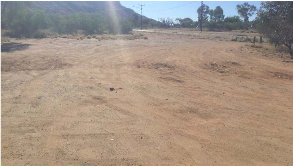
Figure 9 Carpark, condition: poor
