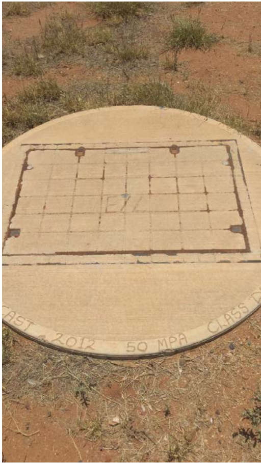
Figure 1 Sewer manhole, condition: excellent
