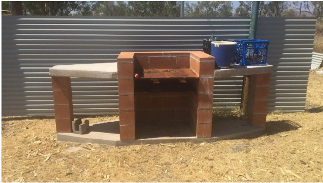
Figure 12 BBQ area, condition: good
