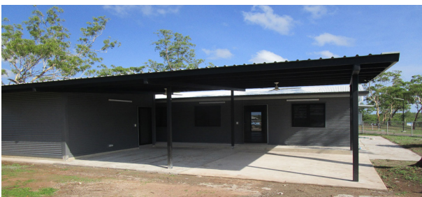
YRAHC sub-contracted Dice (Aust) Pty Ltd to refurbish a previously uninhabitable shelter into a modern four bedroom house.
