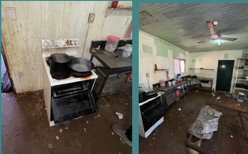
Before works commenced:
