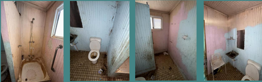
Before Bathroom & Toilet works commenced:
