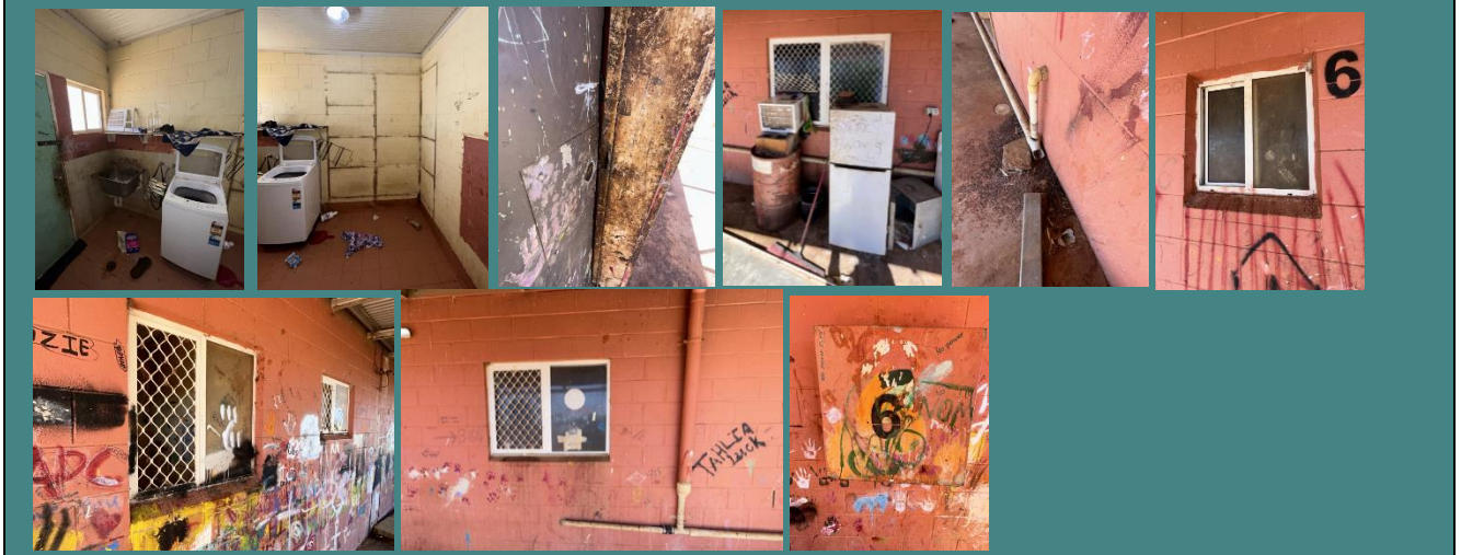
Before Laundry & Exterior works commenced:
