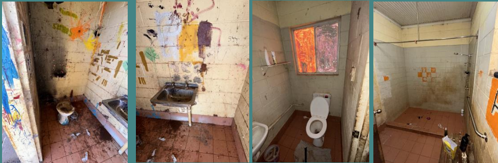
Before Bathroom & Toilet works commenced:
