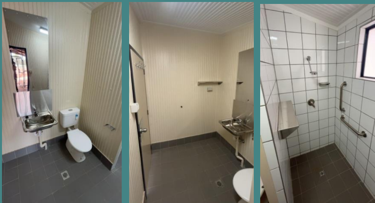
After Bathroom & Toilet works commenced:
