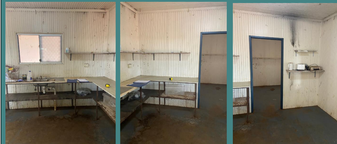
Before works commenced:
