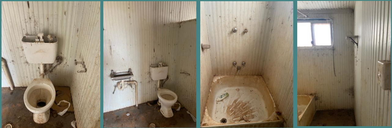
Before Bathroom & Toilet works commenced:
