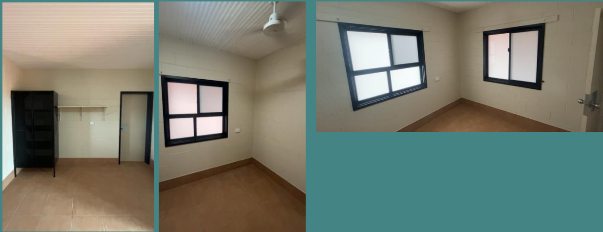
After Bedrooms works completed:
