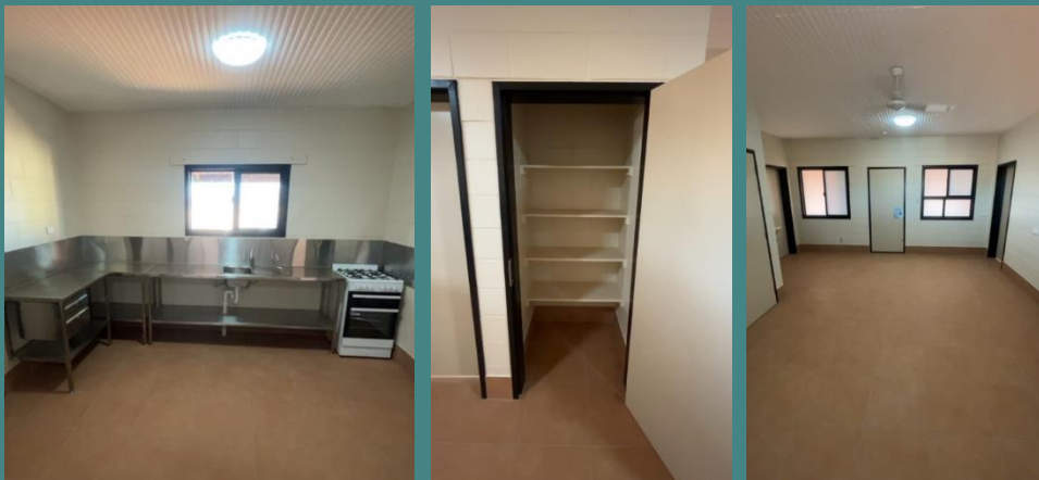
After works completed:
