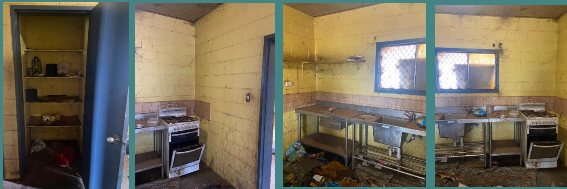
Before works commenced:
