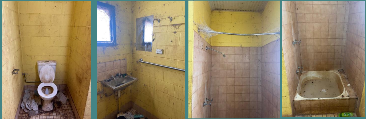
Before Bathroom & Toilet works commenced:
