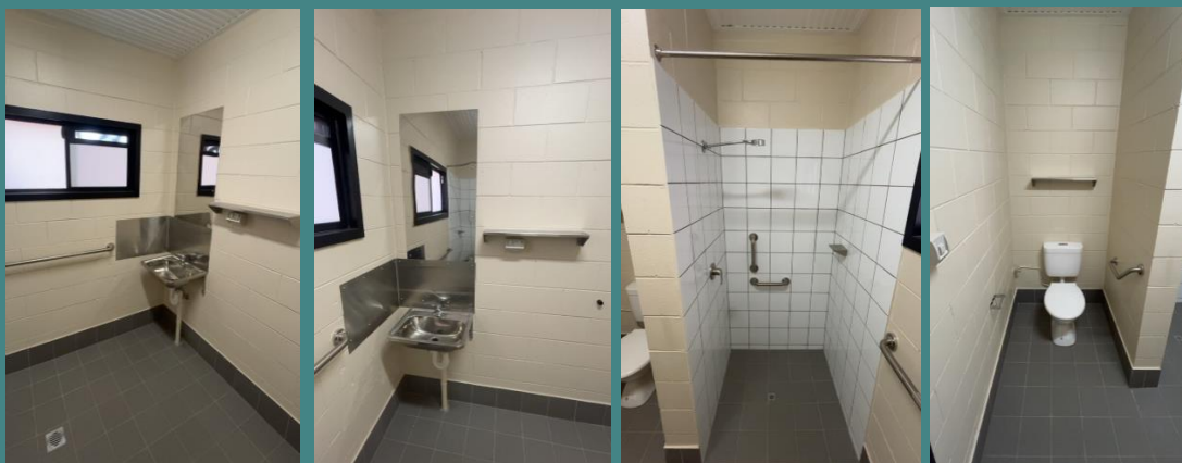
After Bathroom & Toilet works commenced:
