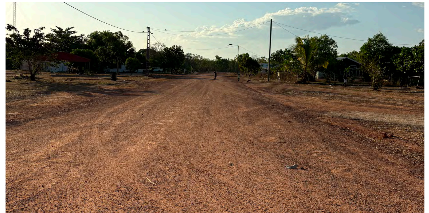
Completed road upgrade, internal road running east/ west
