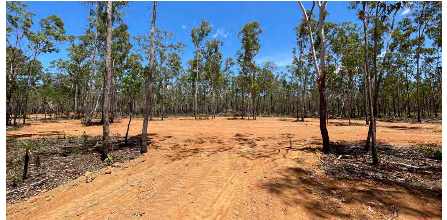
Contractors camp building pad and clearing
