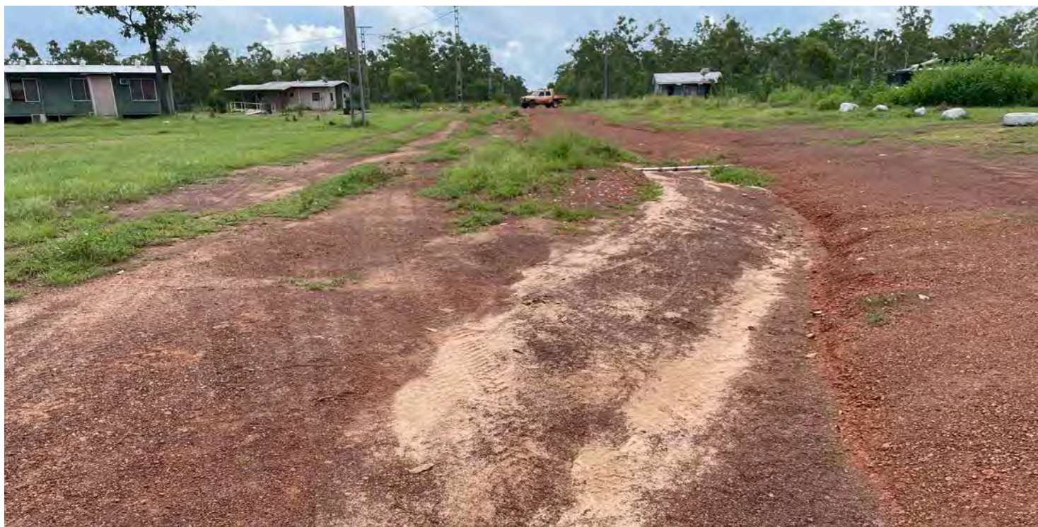
Before photo of internal road running east/ west
