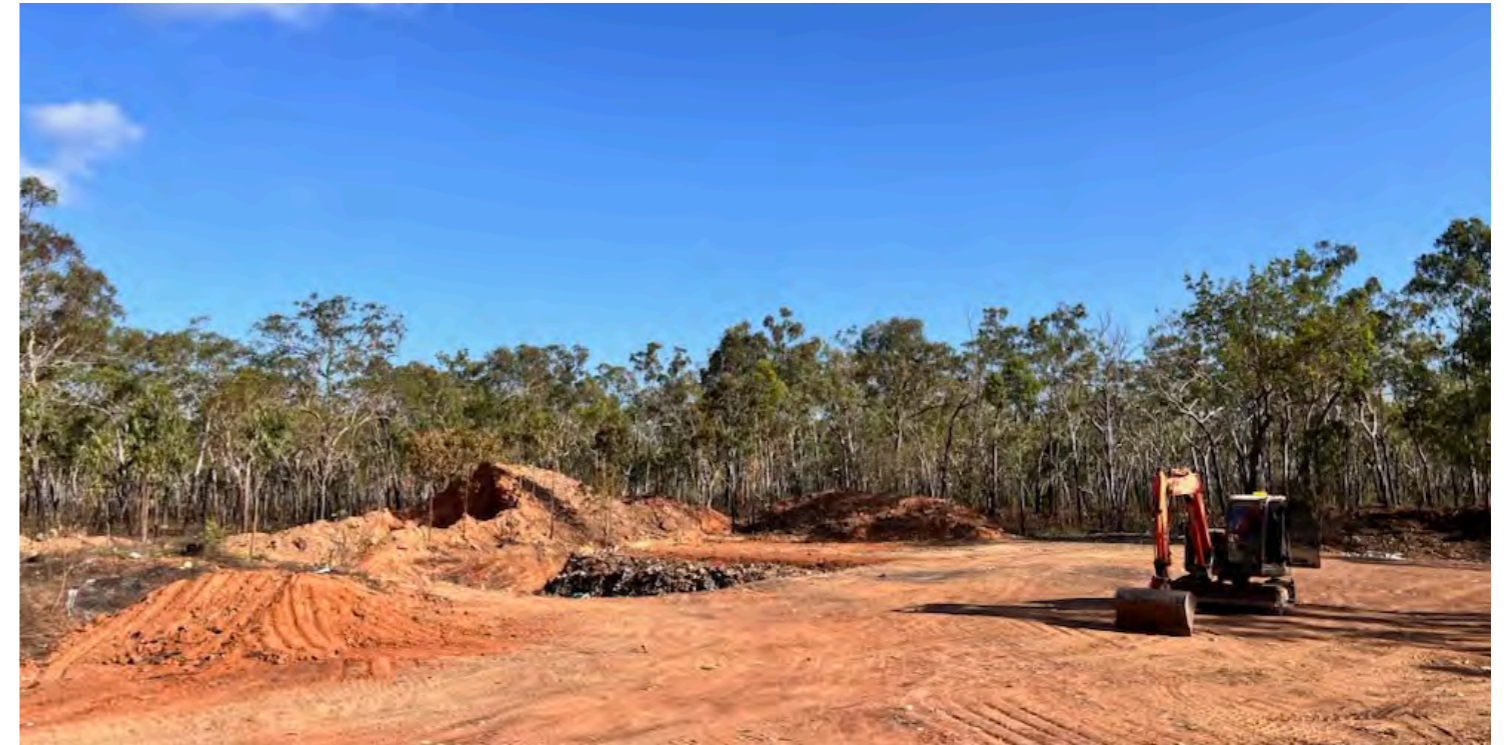
Existing dump capped, dump at ninety-percent capacity
