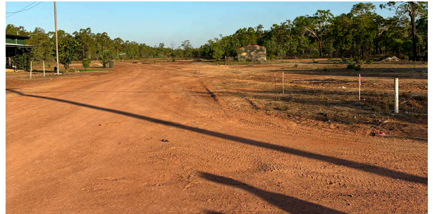
Completed road upgrade internal road and main intersection, view towards east
