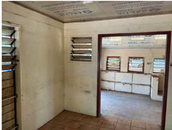
Before – Looking from lounge to kitchen
