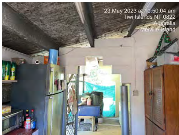
Before – Kitchen to no additional 2 nd bedroom
