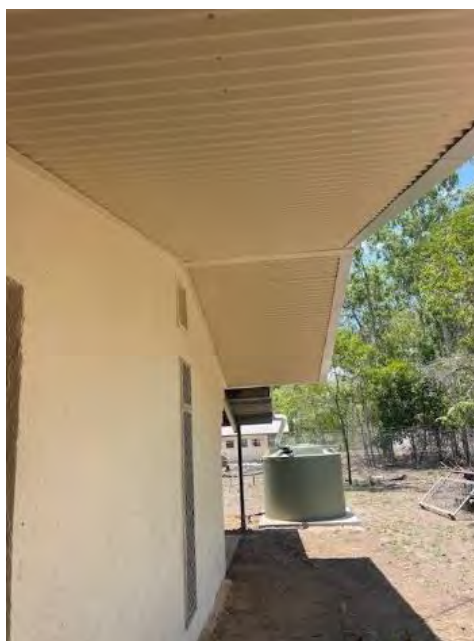
New exterior side shed ceiling
