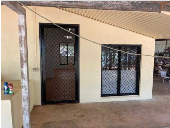
Newly enclosed Area- Outside Front view
