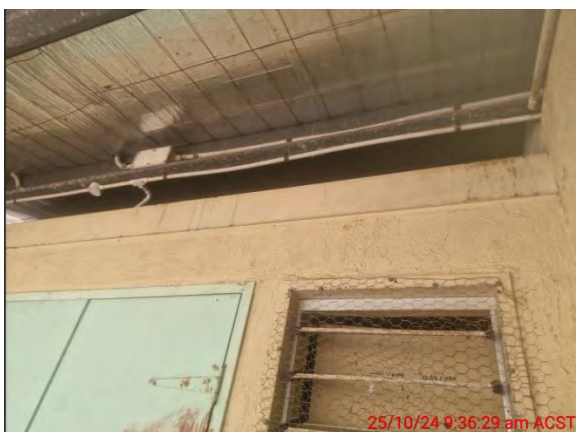
Before paint and ceiling
