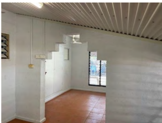
New tiling, paint and ceiling
