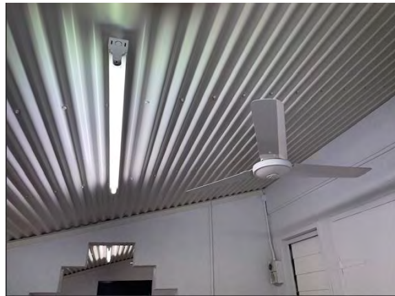
New electricals: Fan and light
